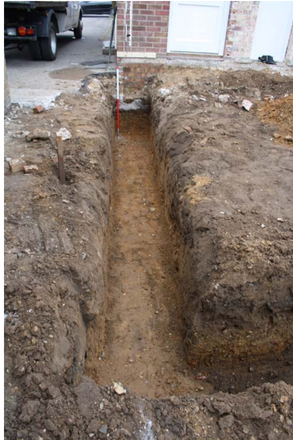
Plate 1. Looking west along south footing trench. Scale 1m.
