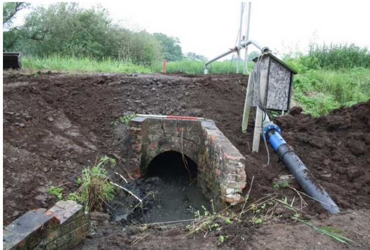
Plate 1. Brick culvert, looking north-west, scale 1m.
