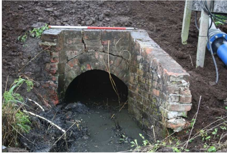
Plate 2. Brick culvert, looking north-west, scale 1m.
