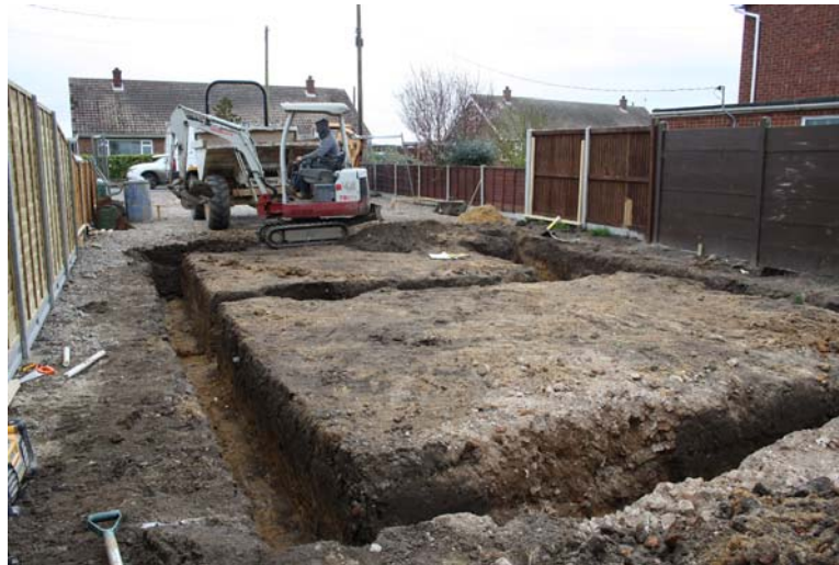
Plate 1. View of site, looking west.
