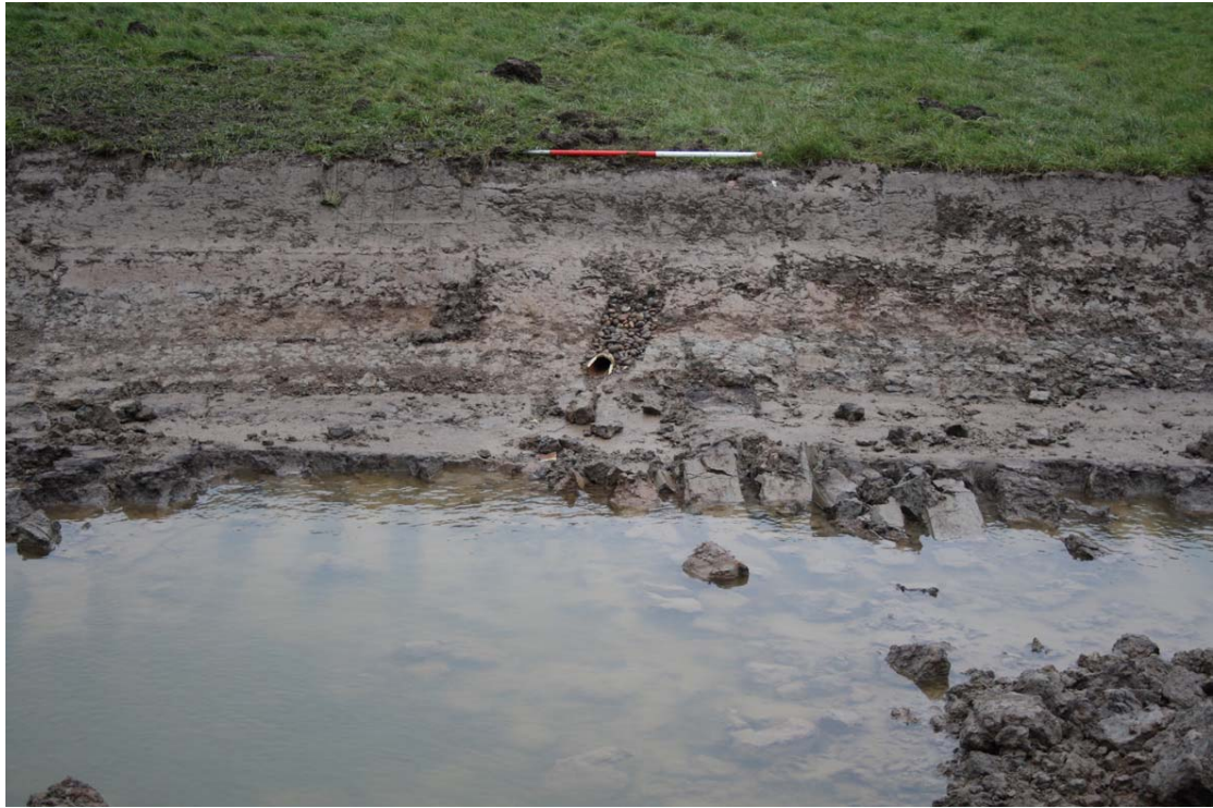
Plate 3. Sourcing of material, typical section with field drain, looking south-east.
