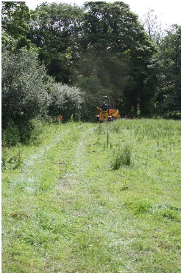
Plate 1. Site at start of works. looking south-east.
