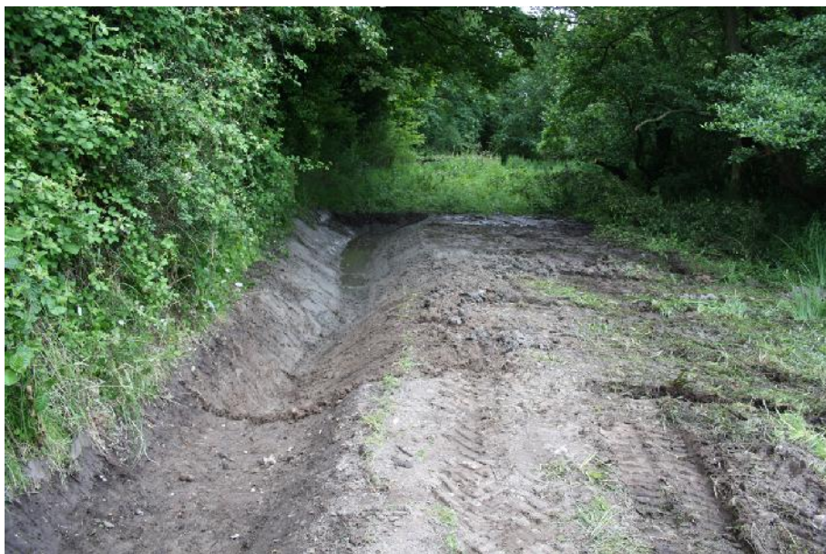
Plate 2. Site at end of works, looking south-east.
