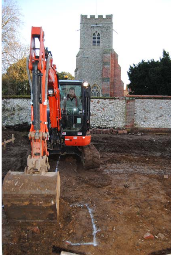
Plate 1 View at start of works. Looking East.
