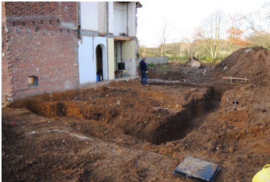
Plate 2 Completed footings. Looking North-West.
