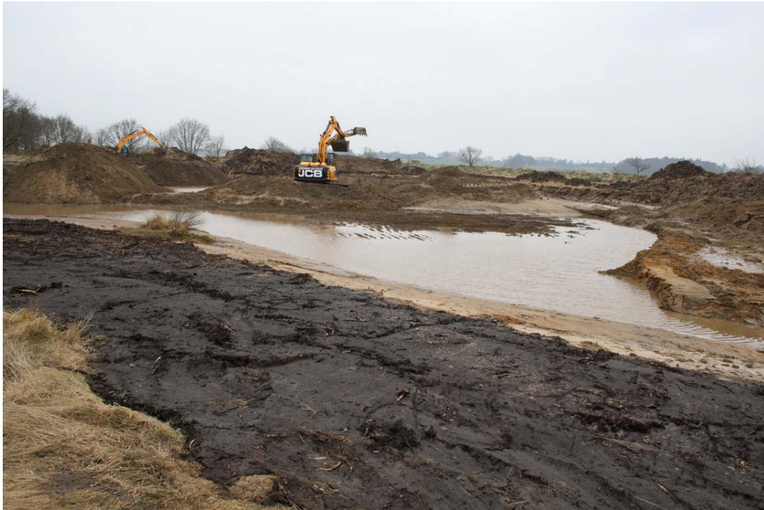
Fig. 3. Excavation of pond, looking north-east.
