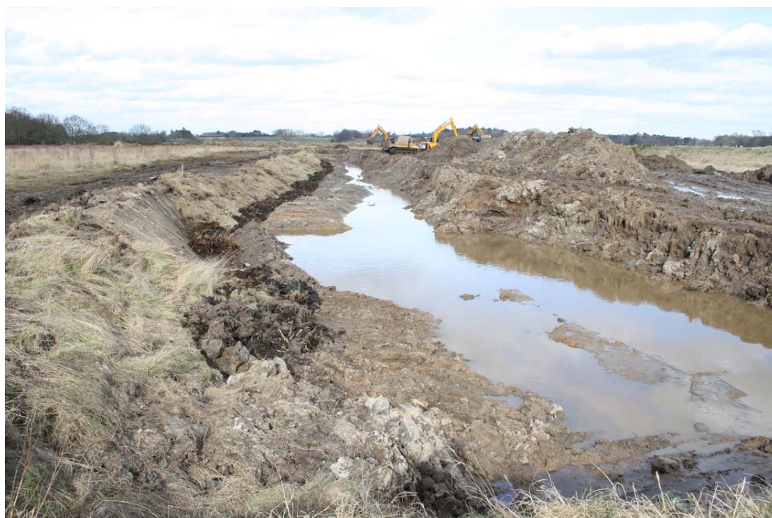
Fig. 2. Excavation of dyke, looking north.
