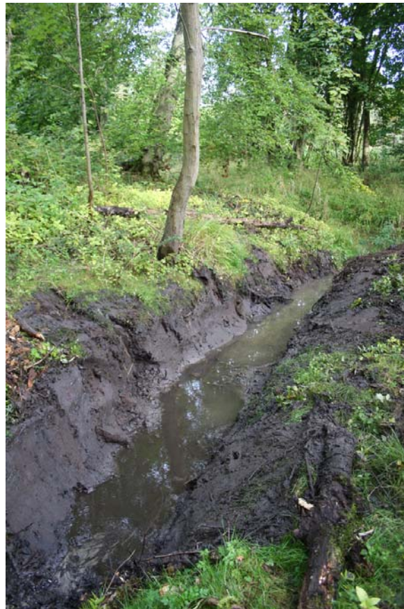
Plate 2. De-silted channel, looking north. Roman Road runs in wooded area to west (left) of channel.
