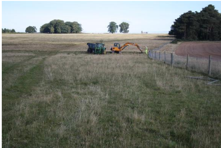
Plate 1. Weeting at start of works, looking North.
