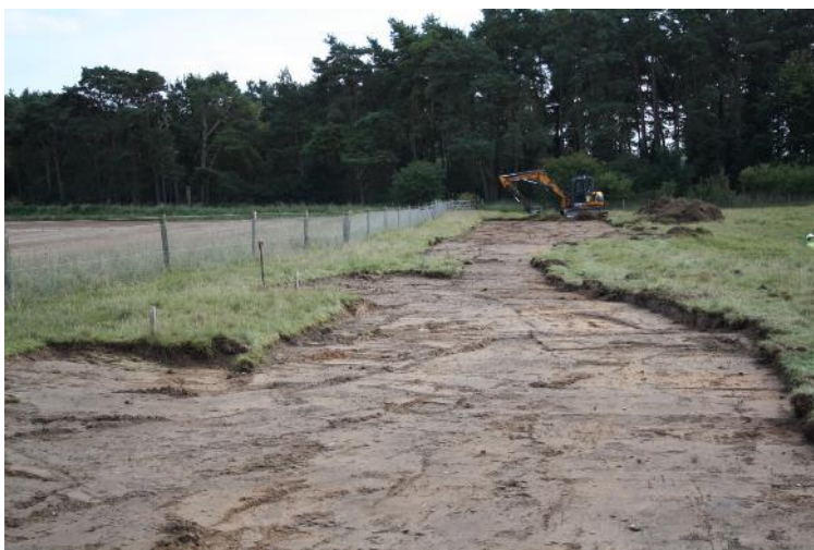
Plate 3. Weeting with works almost complete, looking South
