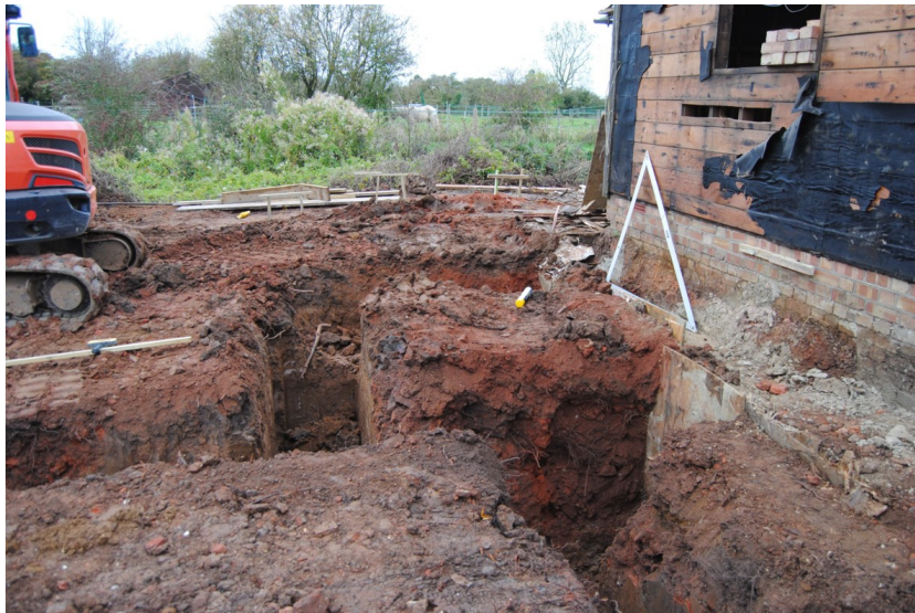
Plate 4. Footing of west extension.
