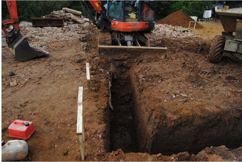
Plate 3. Footing of west extension.
