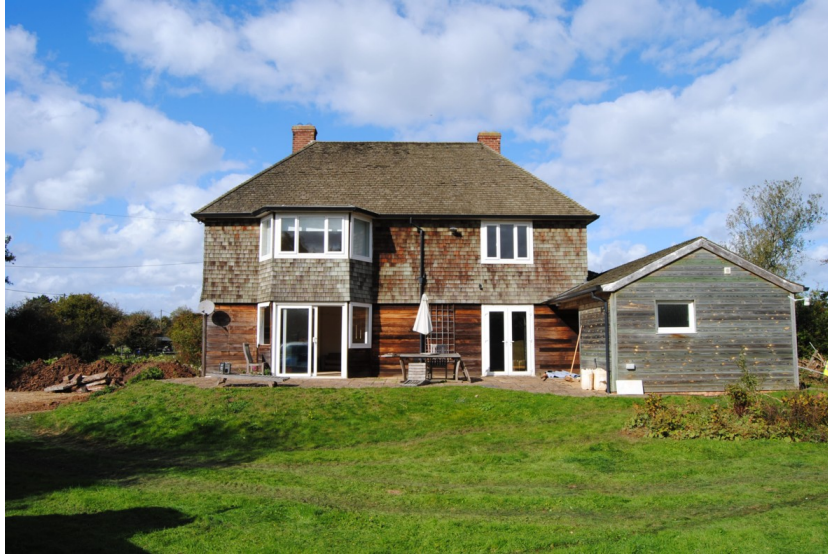
Plate 1. Brook House at start of works.
