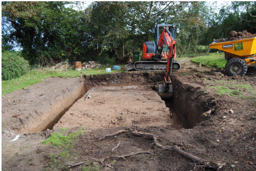
Plate 2. Footings of Workshop.
