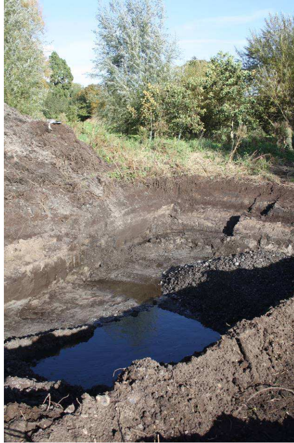
Plate 1. Borrow Pit 1. Feature (08) in section. Looking north-east.
