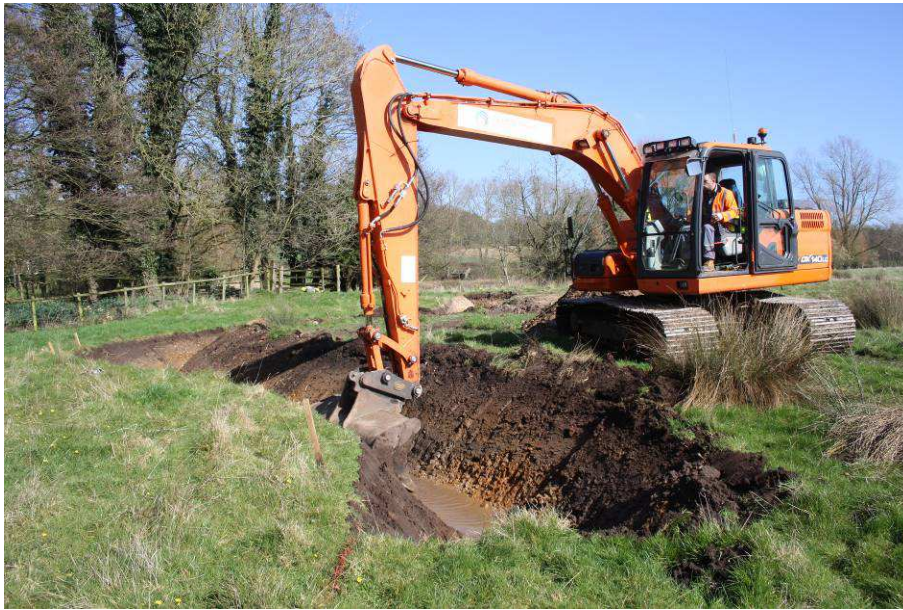
Plate 3. New channel. View of works. Looking north-east.
