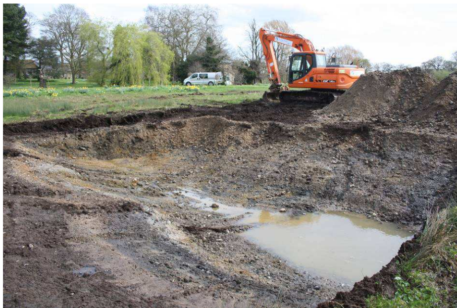
Plate 2. Borrow Pit 3. Looking north-east.
