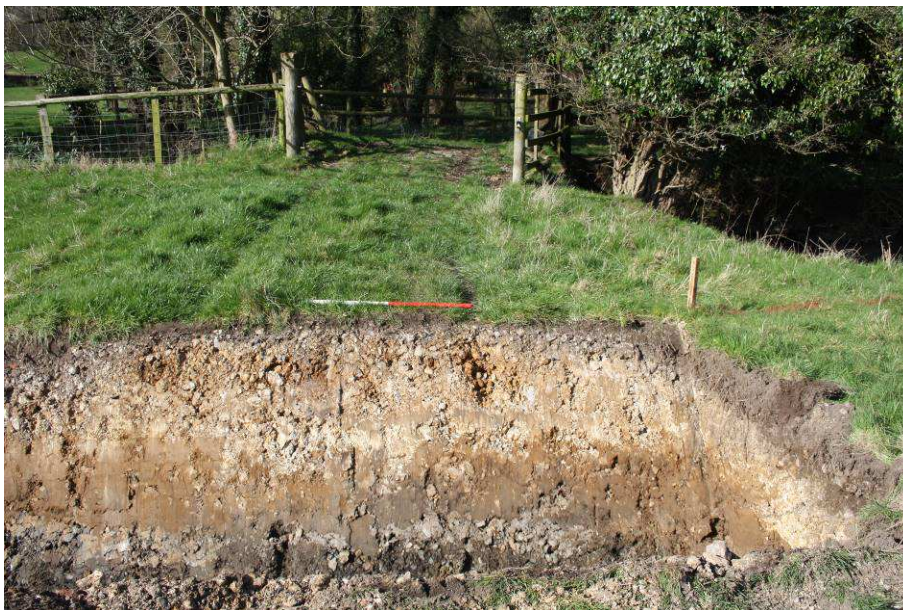
Plate 4. New channel. Section through track. Looking north-west. (Opposite Section A)
