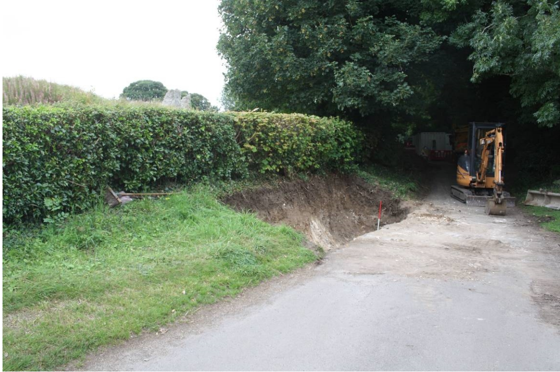
Plate 1. Showing location of soakaway, looking south-west.
