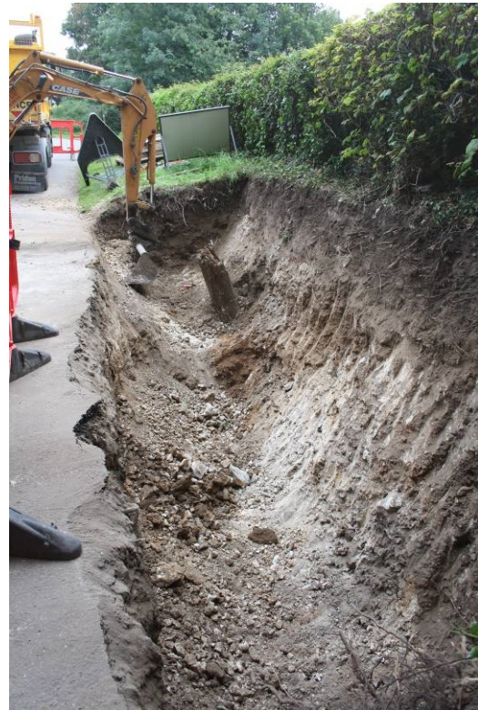
Plate 3. Works in progress, looking east.
