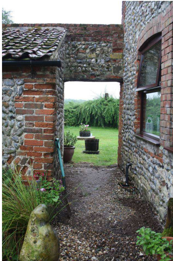
Plate 1. Area prior to works, looking south-east
