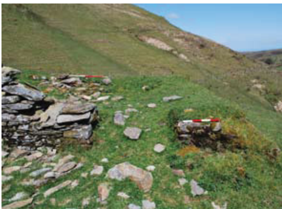
from top Fig 8 Buttress on NW wall Building A Fig 9 NE wall of Building A Fig 10 NW wall Building A Fig 11 Building B
