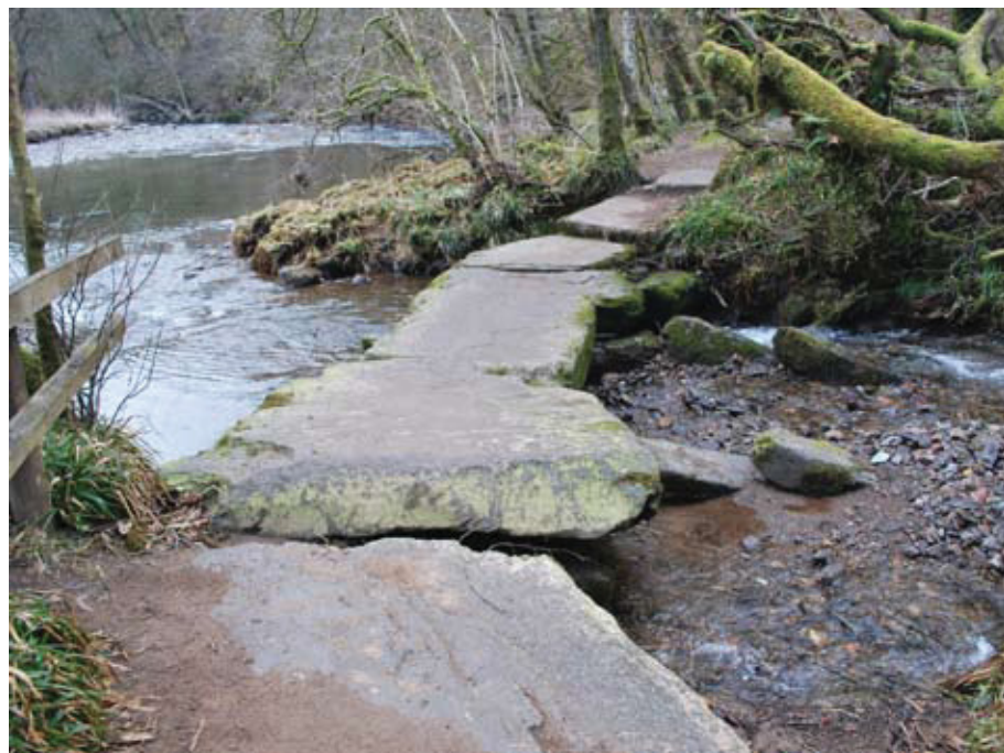
Fig 3 Clapper bridge across West Water at its confluence with the Barle (19/3/2013) (Hazel Riley)
