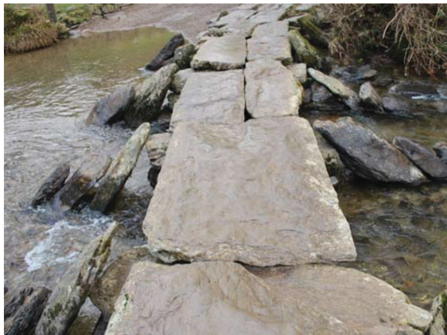
Fig 7 Single and double spans of clapper stones at the Dulverton side of Tarr Steps (19/3/2013) (Hazel Riley)
