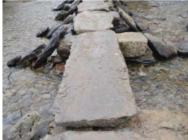
Fig 21 (left) Tarr Steps in the early 20th century (Alfred Vowles) (SRO A/BMS Box 1 T615)
