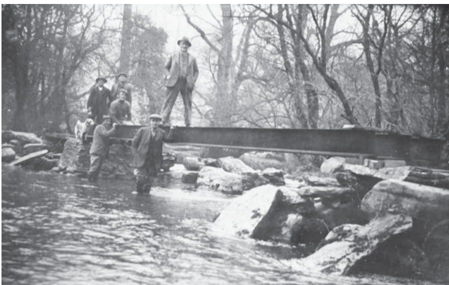
Fig 26 Steel girder and concrete repairs, March 1941 (SRO county neg no 34308)
