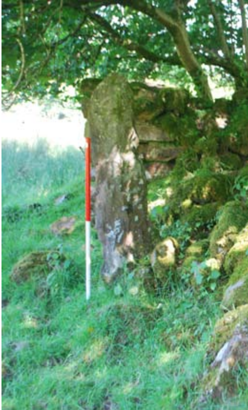
Fig 48 (below) Drain to take water through stone-faced field bank, Bank Down (HCM160149) (Hazel Riley)
