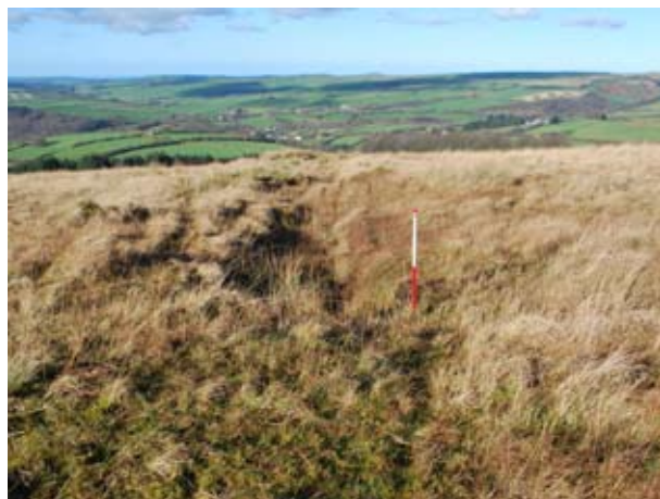
Fig 17 (right) Drainage ditch (CSR17010) on South Regis Common, marked for blocking (1m scale) (Hazel Riley)
