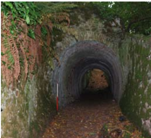
Fig 43 (below) East end of Tunnel 1 (1m scale) (Hazel Riley)
