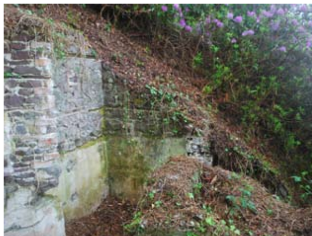
Fig 52 Vegetation clearance from the bath house (Hazel Riley)
