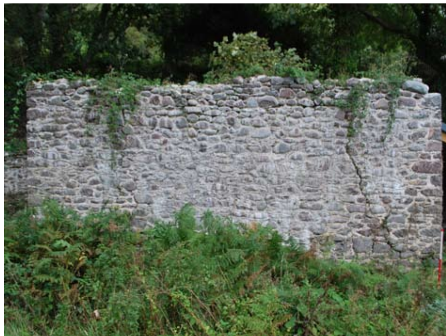
Fig 10 (below) The NE wall of the limekiln (1m scale) (Hazel Riley)
