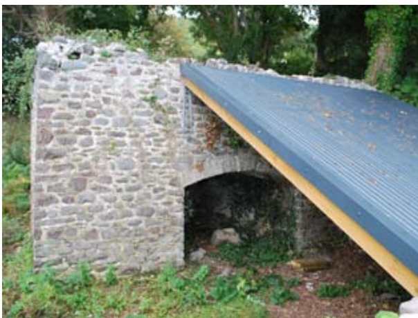
Fig 11 (left) Draw hole access tunnel in NW wall (Hazel Riley)
