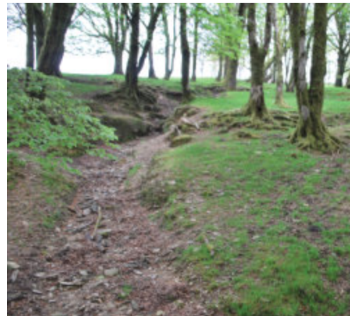
Fig 66 Drainage channels at Clovenrocks Bridge
