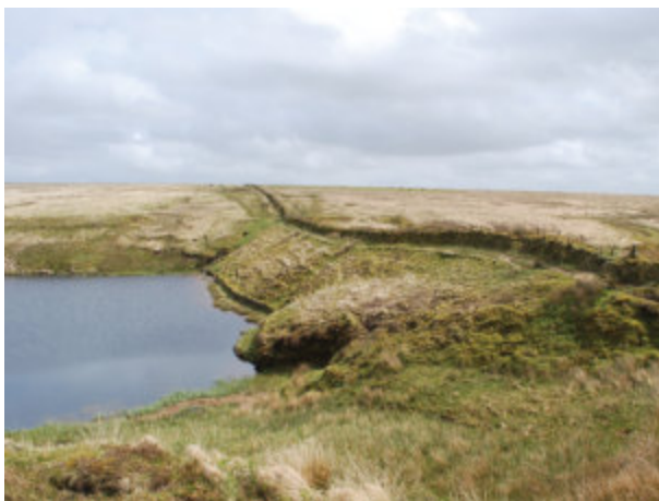
Fig 30 (left) Pinkery Pond and dam: reservoir built to supply water to the Pinkery Canal (Hazel Riley)
