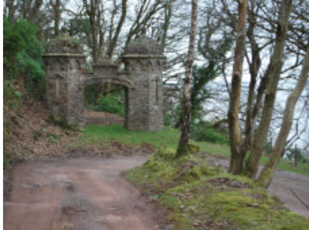
Fig 19 The hairpin bend at The Towers on the main drive to Glenthorne House (Hazel Riley)
