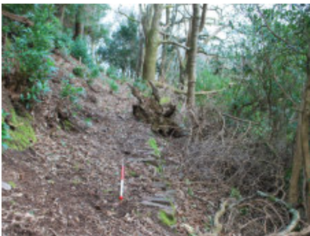
Fig 16 (below right) Detail of retaining wall (1m scale) (Hazel Riley)
