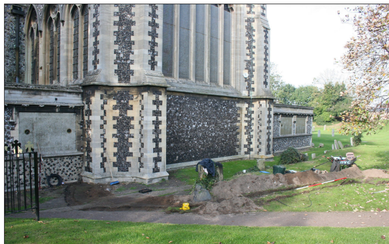
Plate 3: Cable trench position (looking NW) [1x2m Scale]
