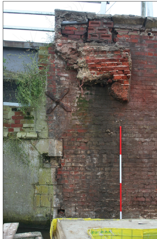
Plate 6: Exposed bridge fabric (looking SE) [1x2m Scale]
