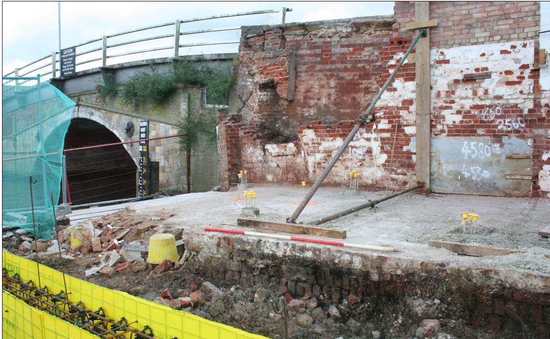
Plate 4: Brick Raft (04) below C19th building (looking SE) [1x2m Scale]
