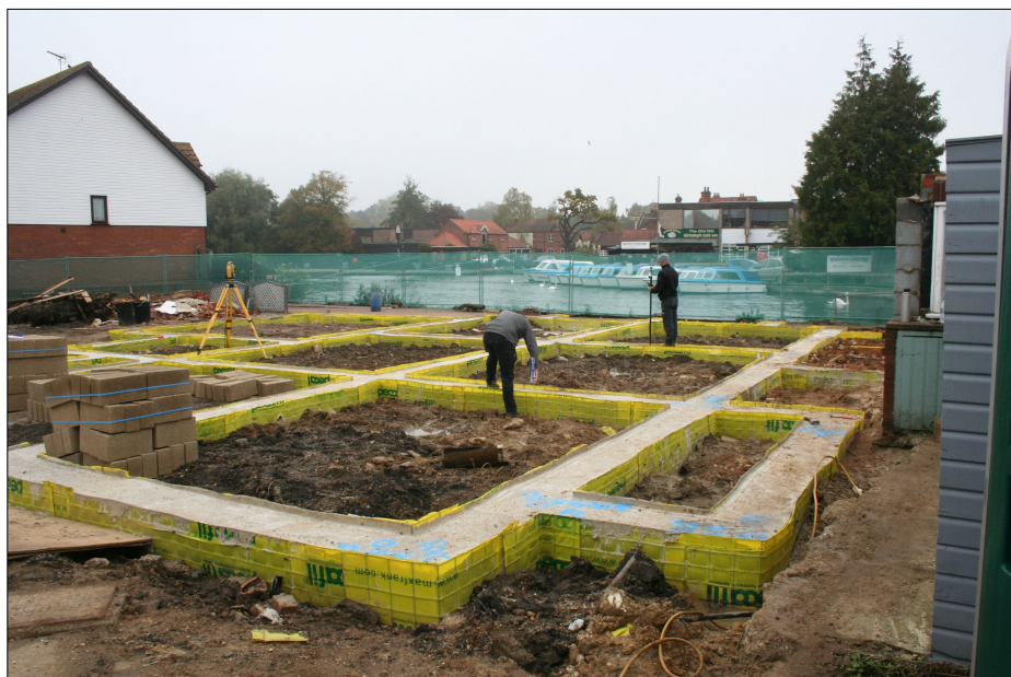
Plate 2: Completed footings (looking NE)
