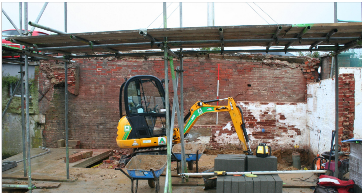
Plate 5: Exposed bridge fabric (looking SE) [1x2m Scale]
