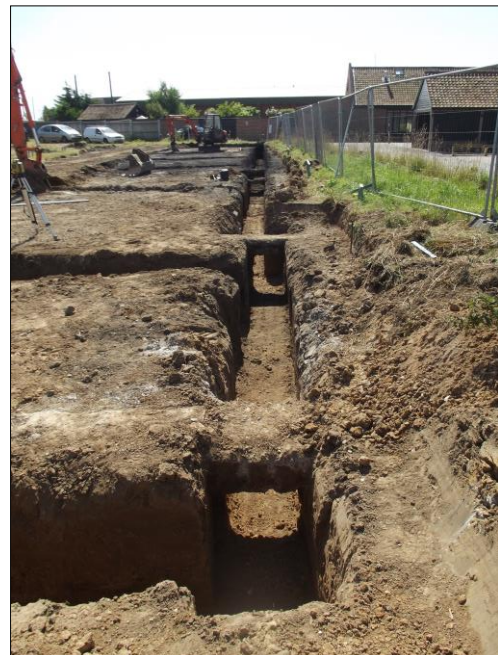
Plate 2. General footing trench shot (looking SSE)
