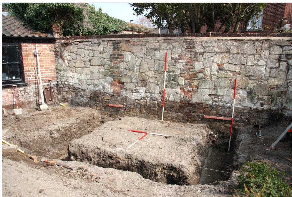
Plate 3. Footing trenches (post-machining), looking east [2x2m & 2x1m Scales]
