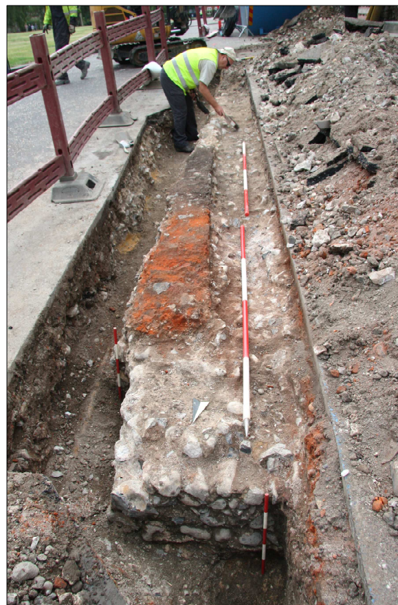
Plate 4. Bell Tower Footings. (Looking S) [10.5m & 2x2m Scales]
