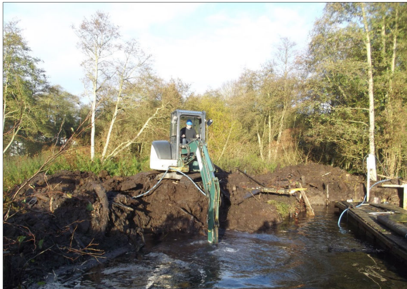
Plate 5: Wet-machine work in the New Basin (NE corner), looking North
