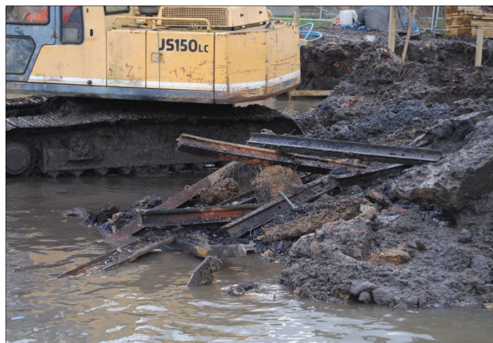
Plate 8: Rails after removal from the Hotel foundations, looking SW
