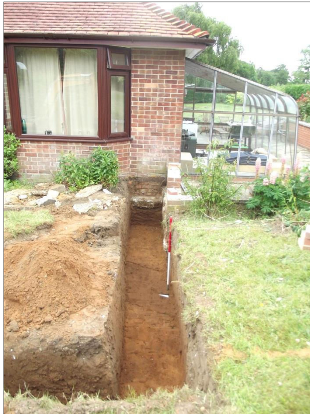
Plate 3: Ditch [04] (looking SE) [1x2m Scale]
