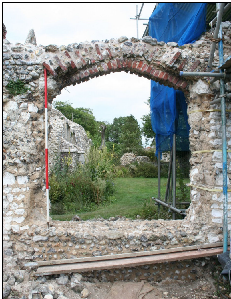
Plate 4: Window 1 (S. Elevation) [1x2m Scale]
