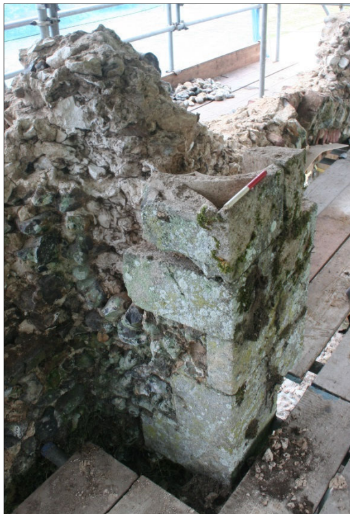
Plate 17: Reused Decorative Masonry (looking SW) [1x0,2m Scale]
