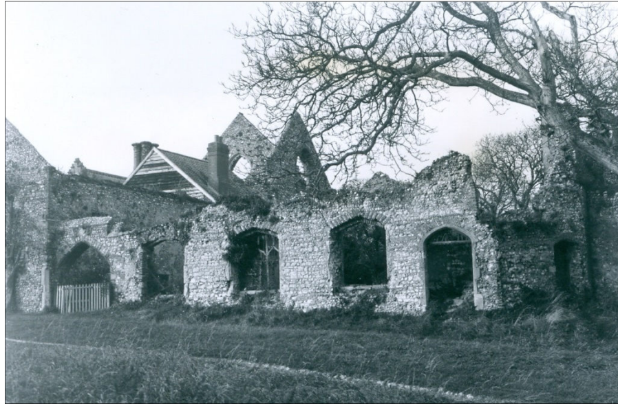
Plate 2: South Elevation of the S. Range taken in 1954 (H.G.Thursford)
