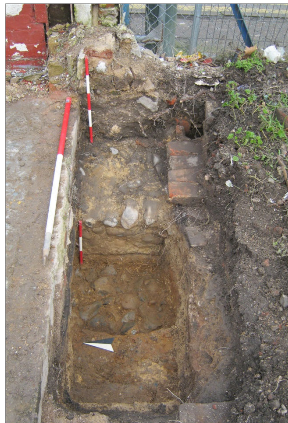
Plate 6: Wall of a medieval building constructed on a flint packed footing trench revealed within the confines of F26. [1x1m, 1x0.5m & 1x0.3m Scales]
