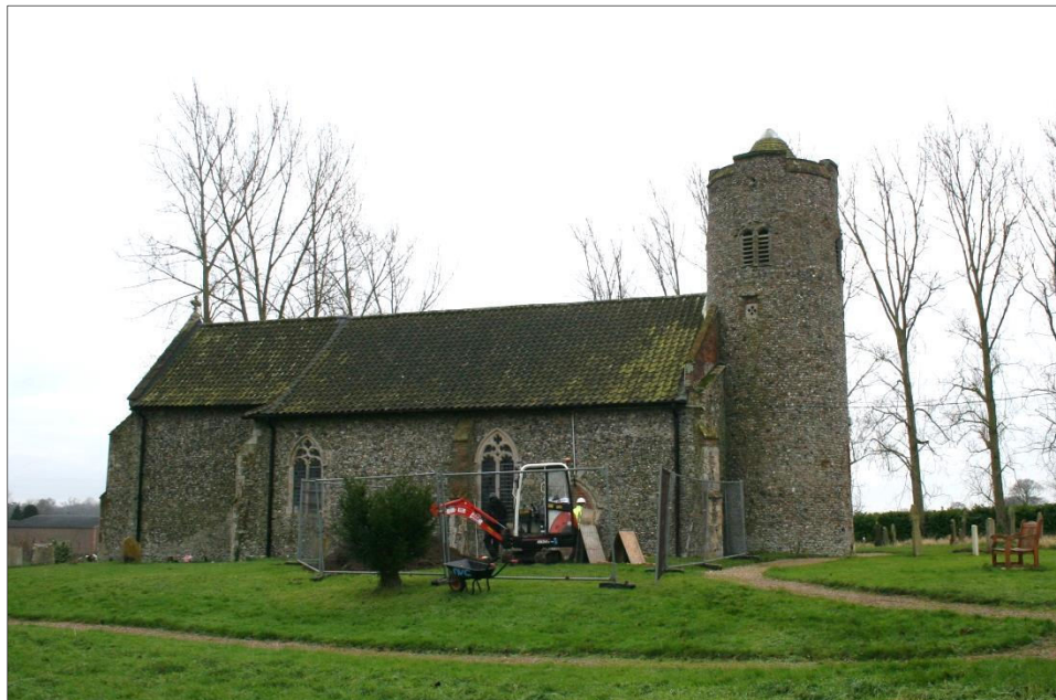
Plate 2: Location shot of the extension works (looking south-east)
