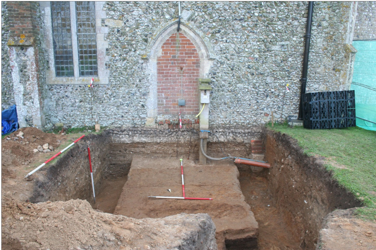
Plate 6: Excavation Area – Post-excavation (looking S) [2x2m & 2x1m Scales]
