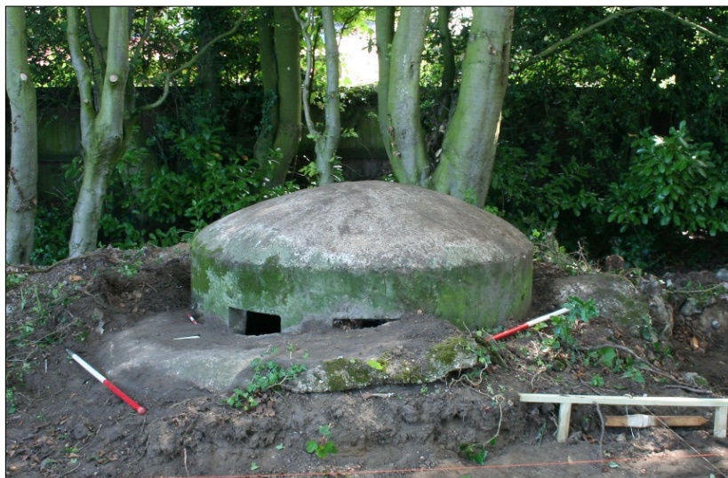
Plate 5: Norcon Pillbox. (looking E) [2x1m scales]
