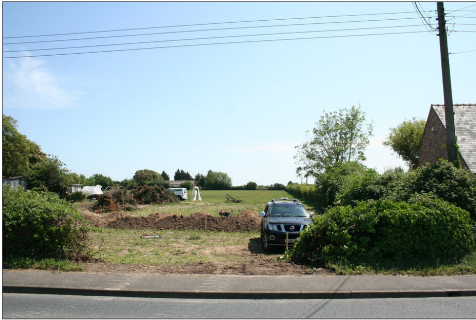
Plate 2: General shot of the site during trench works (looking SE)
