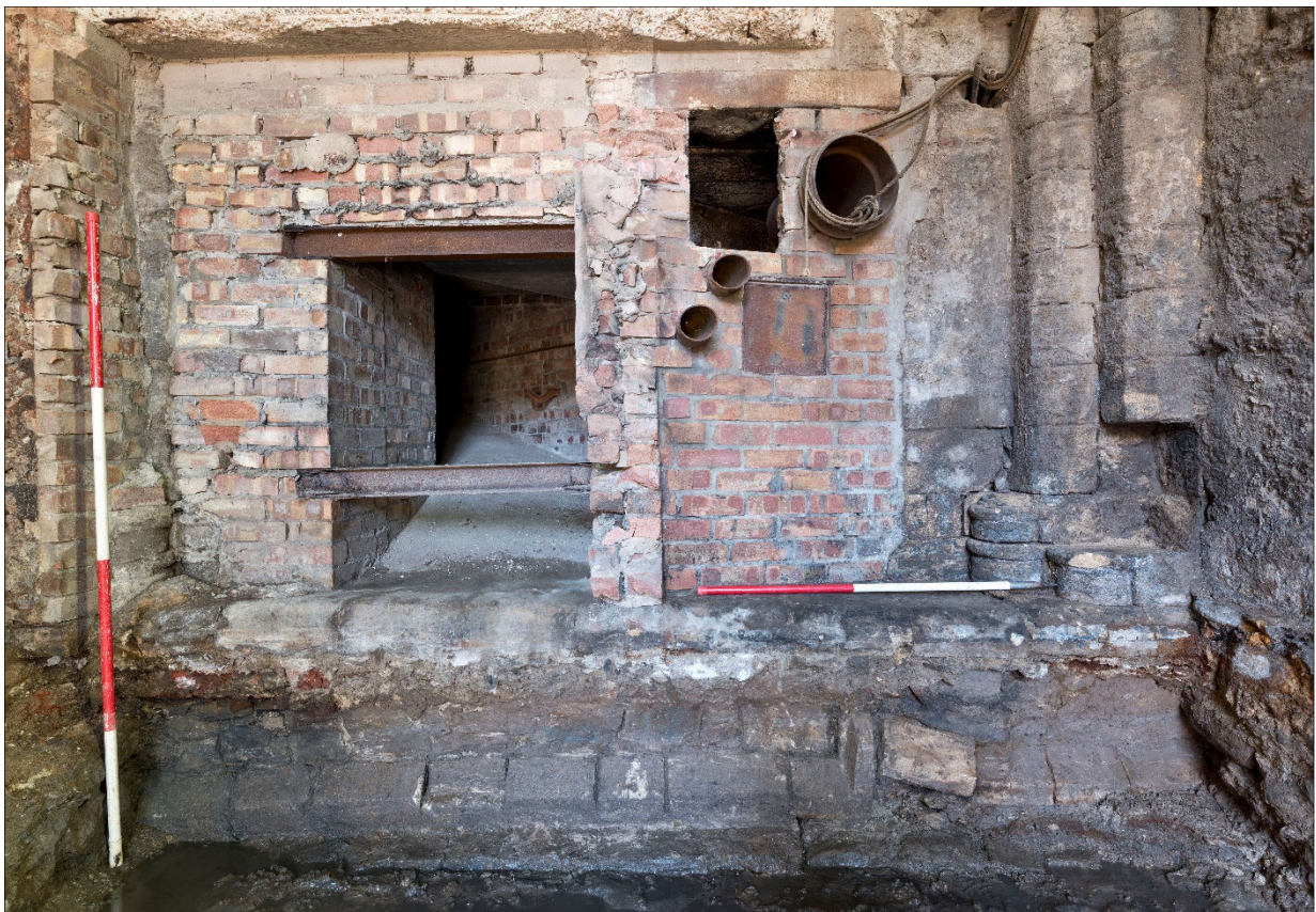
Plate 22: Medieval masonry exposed inside the tower (below the modern concrete floor) (looking E) [1x1m & 1x2m Scales]
