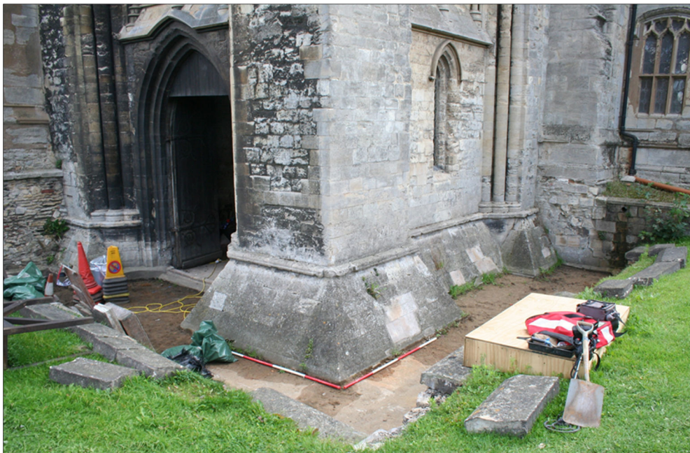
Plate 10: General working shot of moat area (looking NE) [2x2m Scales]
