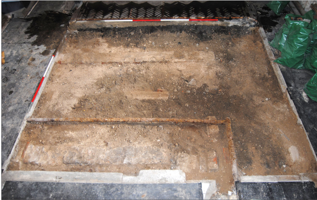
Plate 5: Re-flooring work Area D (looking E) [1x1m & 1x2m scales]
