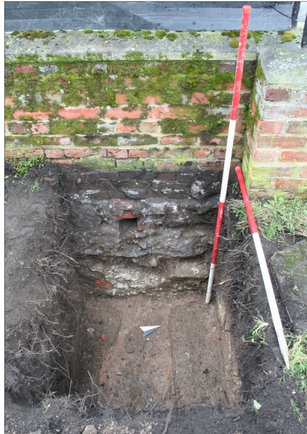
Plate 8: Cable connection trench (looking W) [1x1m & 1x2m scales]
