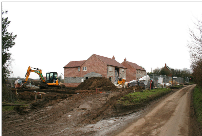
Plate 2. General progress shot, Plot 1 Garage in fore (looking E)
