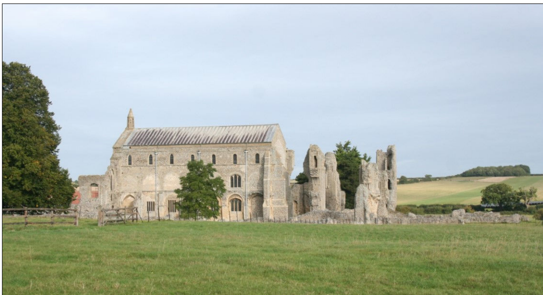
Plate 2. General view of the Priory Church and remains. (looking N)
