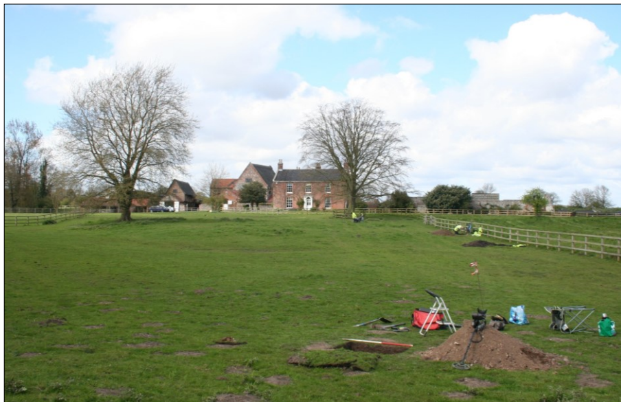
Plate 2. Working shot (TP1 in foreground), looking NNW
