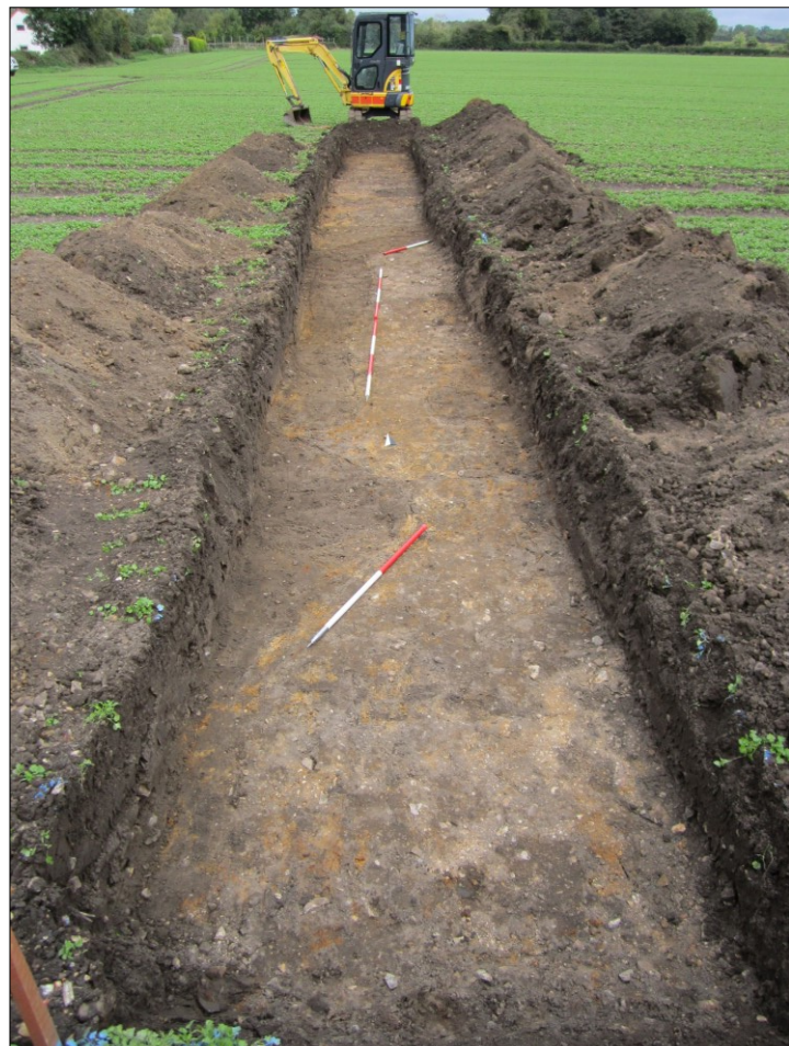
Plate 2. Exposed features. (looking N) [1x1m Scale in foreground]
