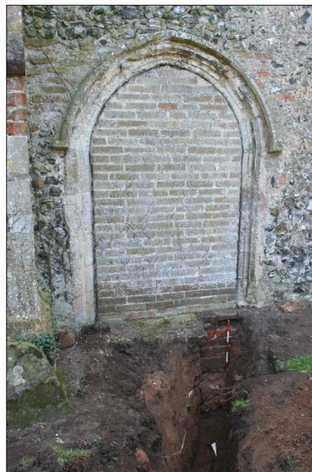
Plate 4. Blocked North Door. (looking S) [1x0.5m]
