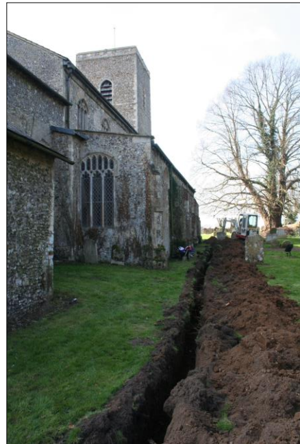
Plate 2. Water pipe trench. (looking W)
