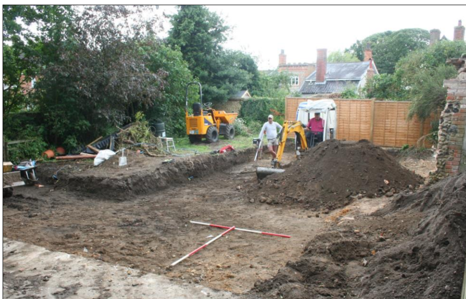
Plate 5. Trench (looking ESE) [2x2m Scales]
