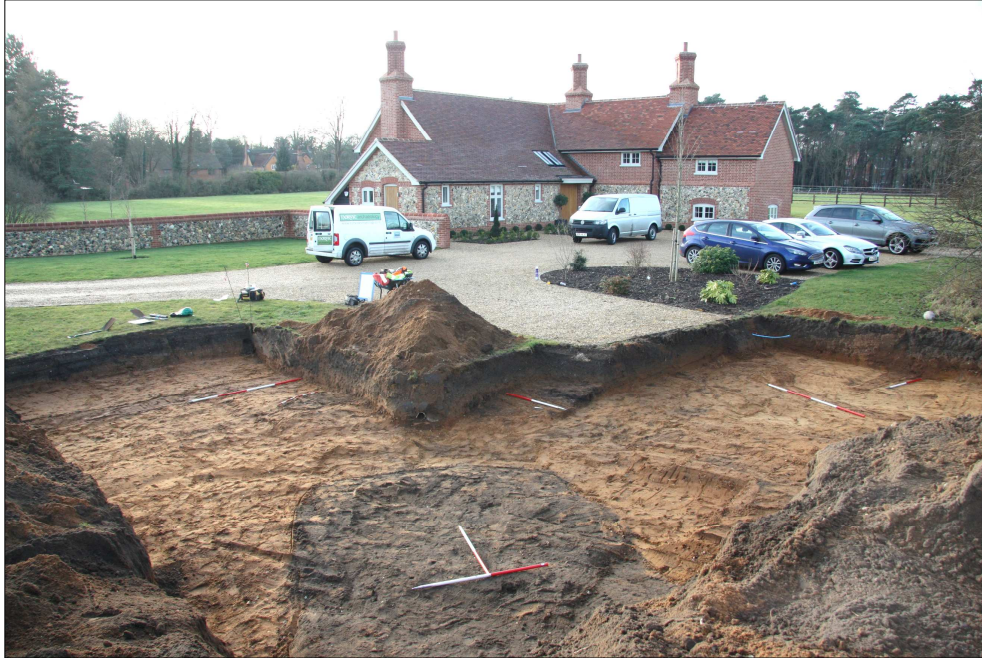
Plate 2. Trench during excavation (looking SW) [Scales shown are either 1m or 2m rods]
