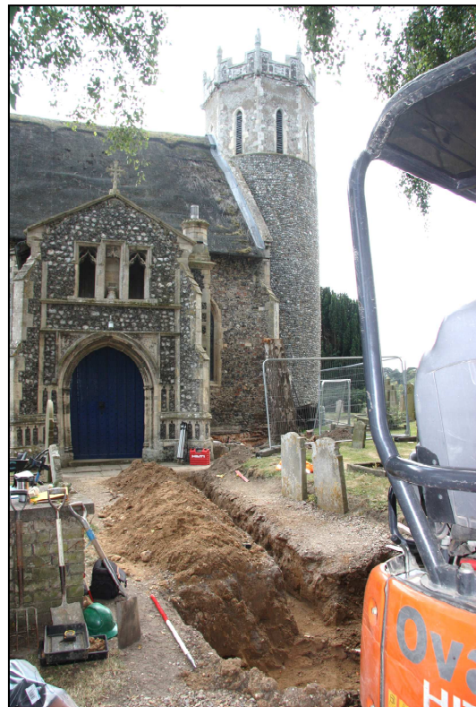
Plate 2. New soakaway and drain trench. (looking SSW) [1x1m Scale]
