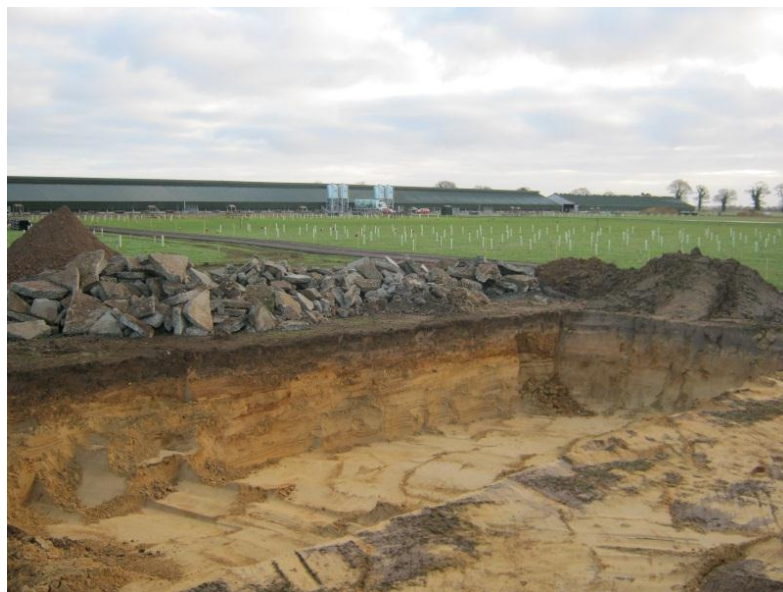
Plate 4: Western Secondary Sump Trench @3m depth (looking east)
