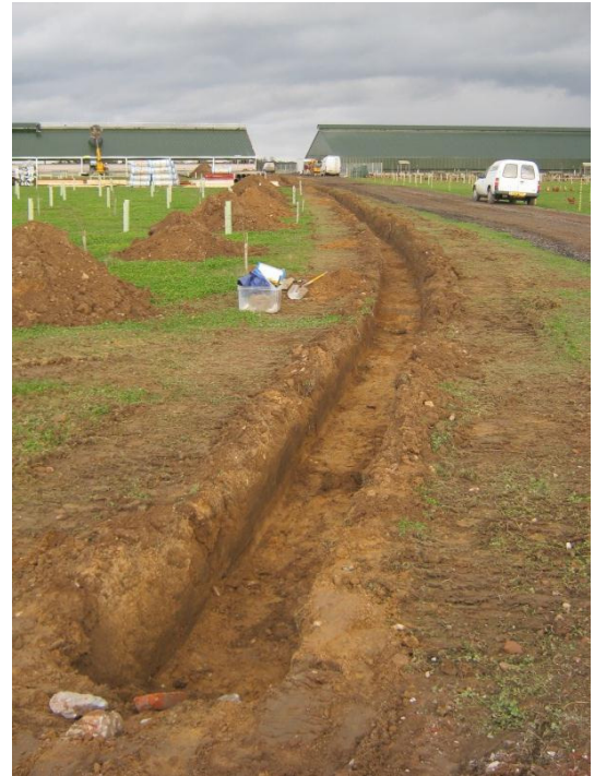
Plate 3: Western drainage trench (looking north-east)
