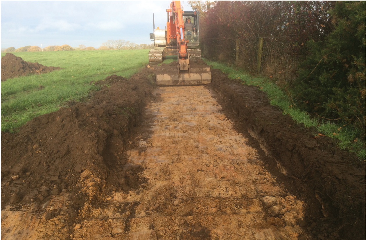
Fig. 3 Light orange glacial till (underlying substrate) is revealed beneath a loamy topsoil
