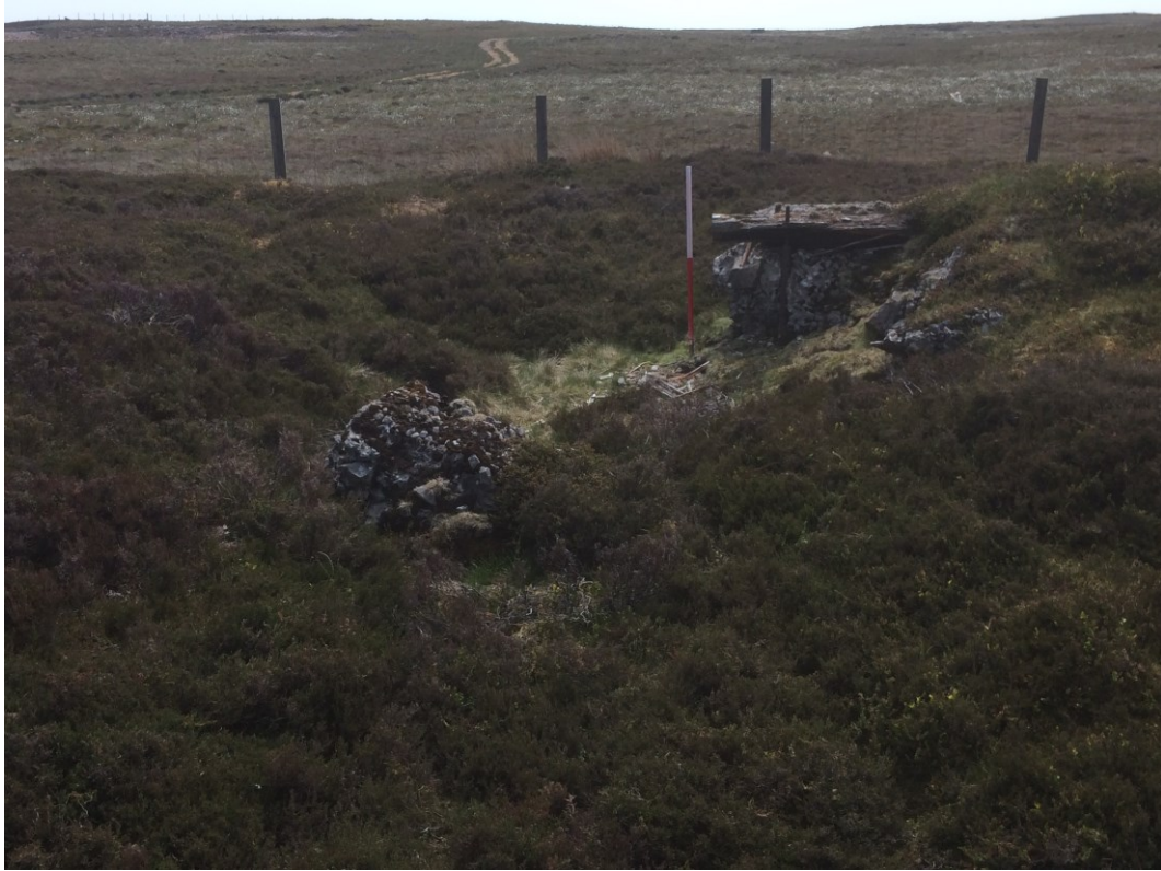
Figure 6 Hollow to the south of the shaft mound still carrying the broken concrete block presumably associated with the early 20th century engine (scale 1m)
