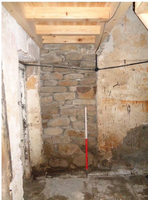
Figure 23 Room G4, facing west. Detail of blocked doorway. Scale 1x1m
