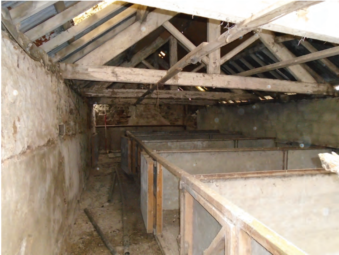
Figure 74 Building B, Room G1, facing south. Scale 1x2 m
