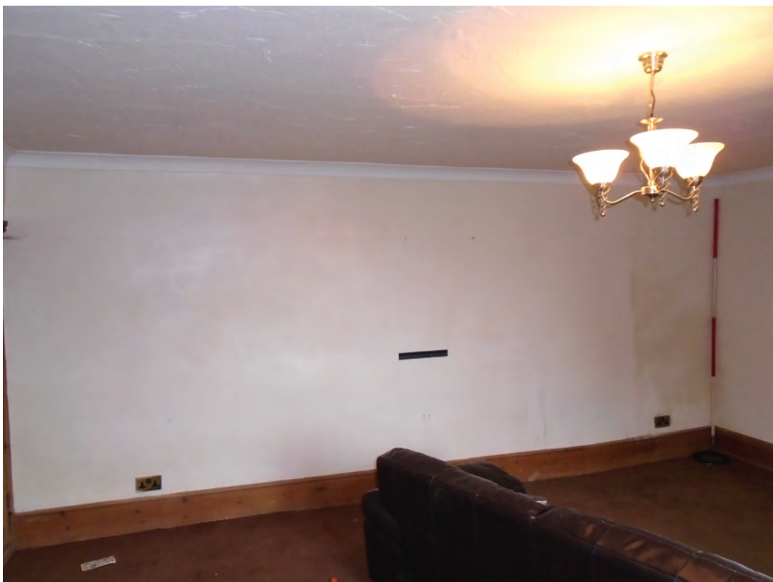
Figure 26 Room G7 facing north-east. Scale 1x2 m
