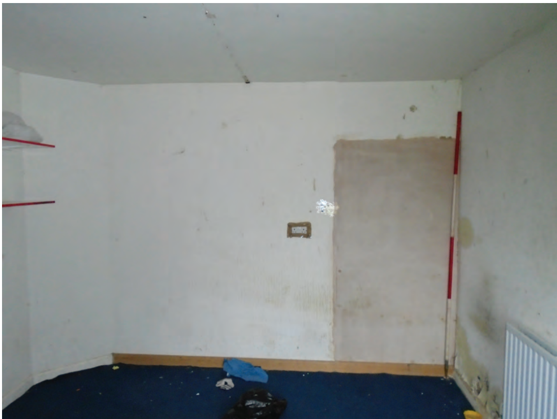
Figure 14 Room G2, looking north. Scale 1x2 m
