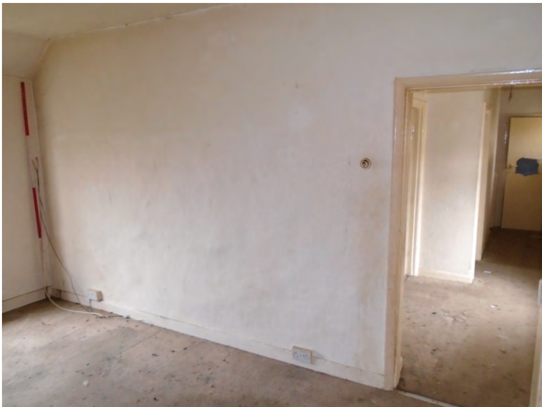
Figure 43 Room F1, facing south-west. Scale 1x2 m
