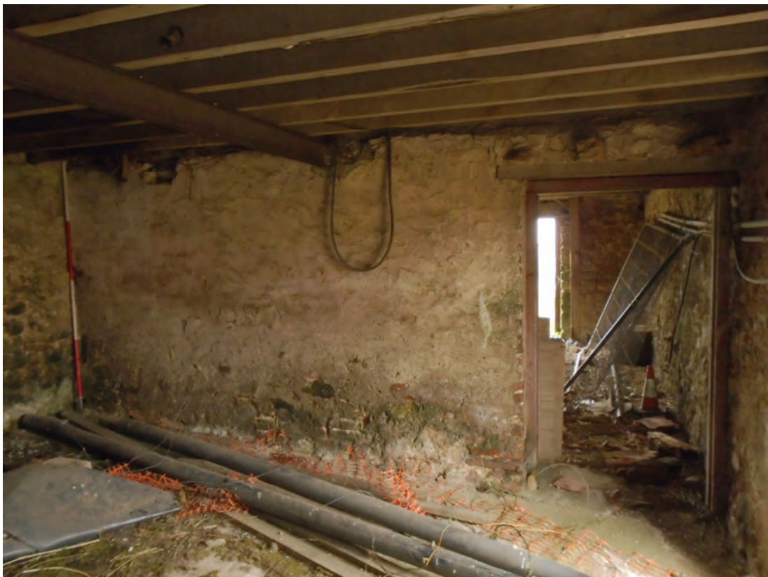
Figure 82 Room G3, facing north-east. Scale 1x2 m
