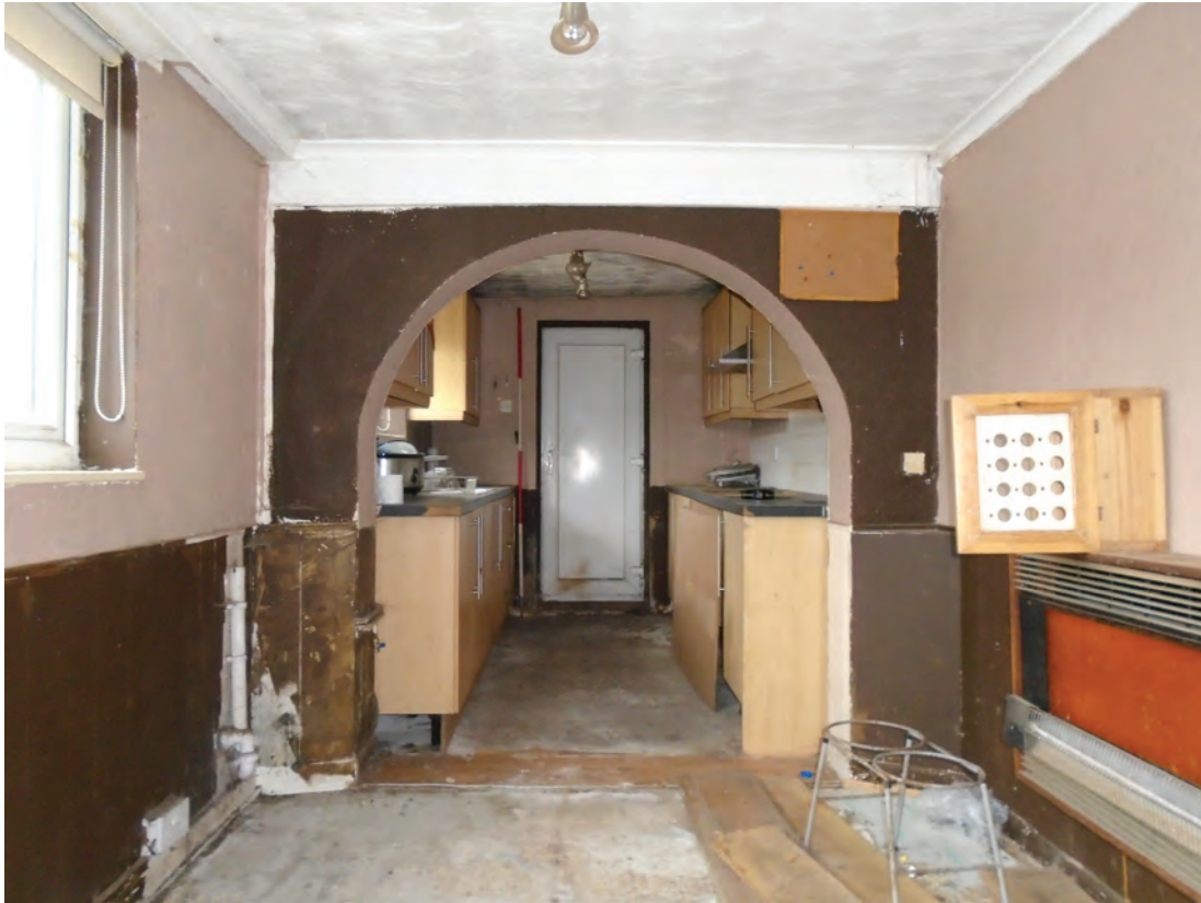
Figure 19 Room G4/G5 facing east. Scale 1x2 m
