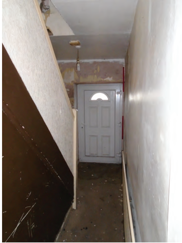
Figure 21 Room G6 looking south. Scale 1x2 m
