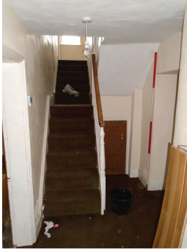
Figure 34 Room G10 looking north. Scale 1x2 m
