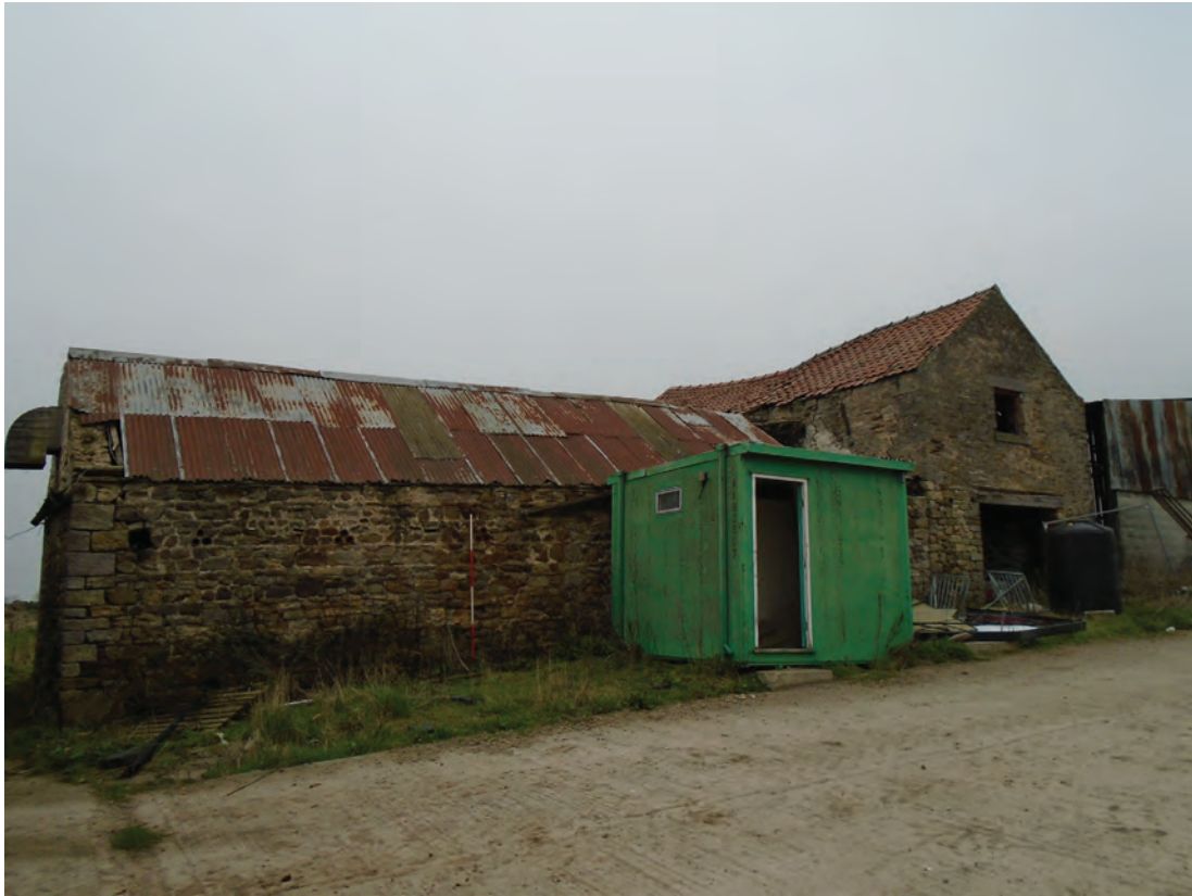
Figure 68 Building B, east elevation, facing north-west. Scale 1x2 m
