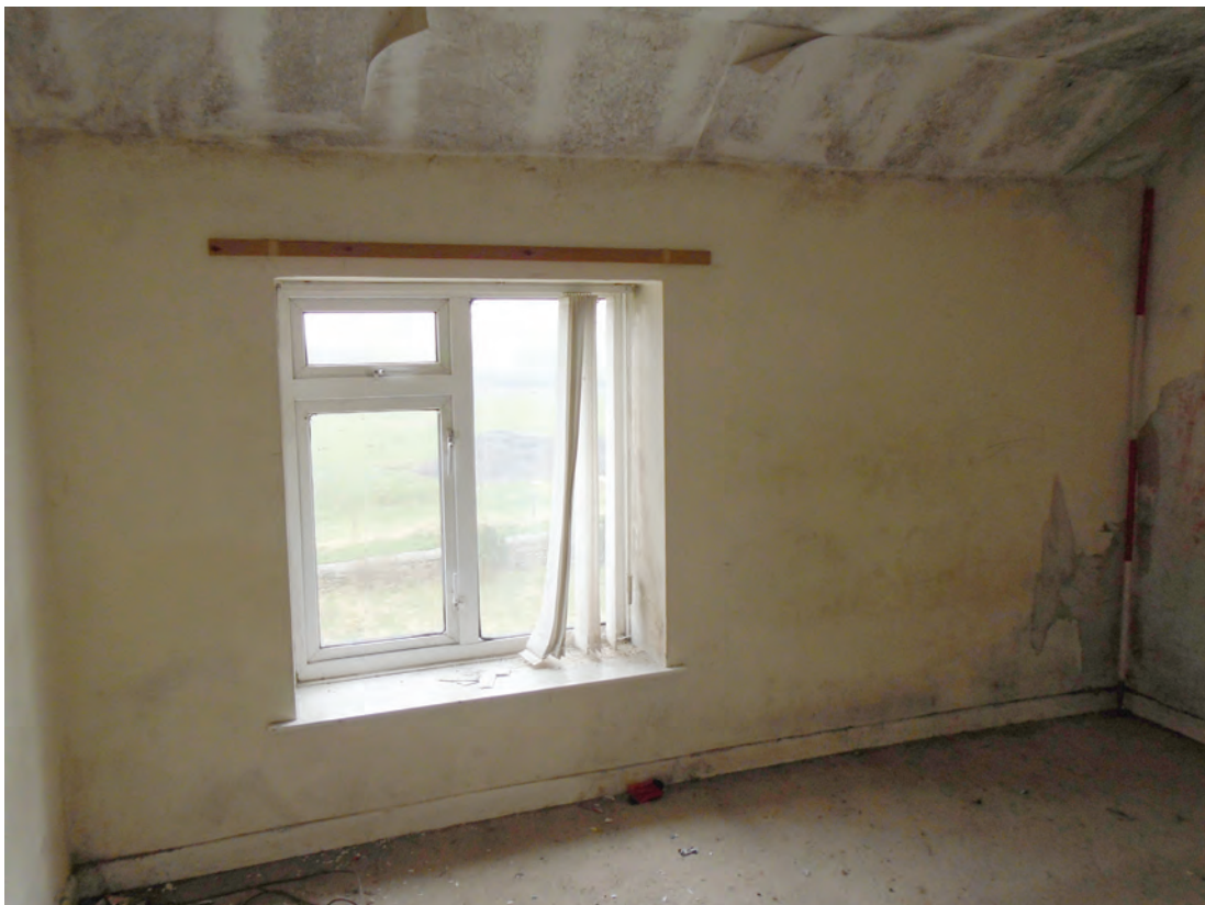
Figure 51 Room F4, facing south. Scale 1x2 m
