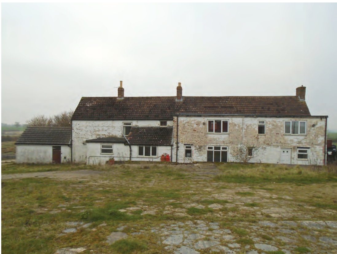
Figure 7 North elevation of Building A, facing south. Scale 2x2 m
