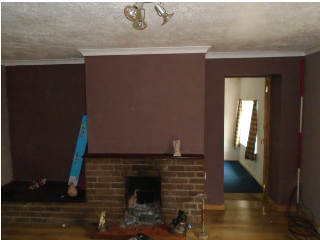
Figure 16 Room G3 looking east. Scale 1x2 m
