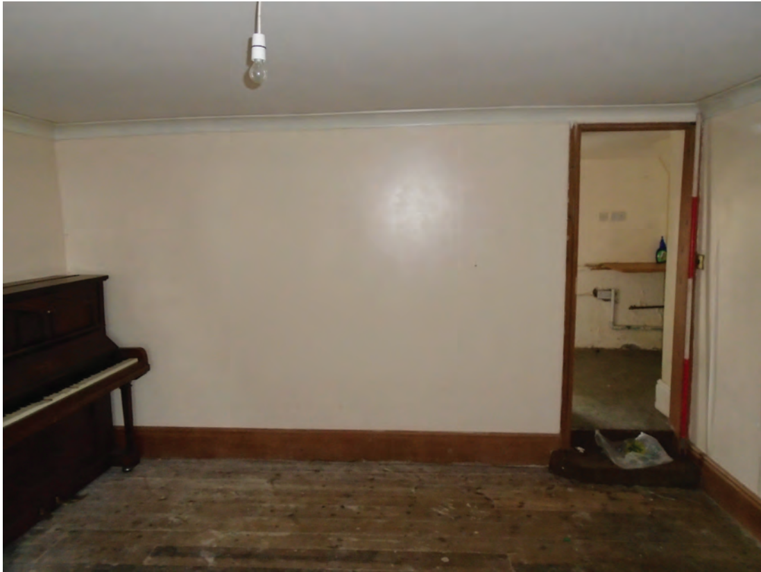
Figure 36 Room G11 looking north. Scale 1x2 m
