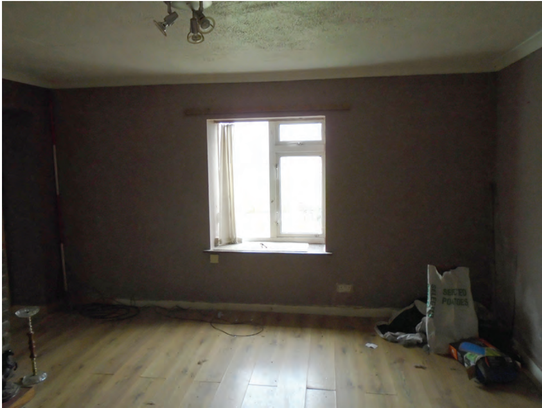
Figure 17 Room G3 looking south. Scale 1x2 m
