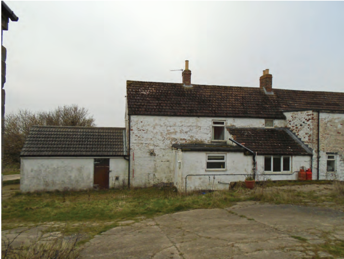
Figure 8 East extent of north elevation of Building A, facing south-west. Scale 2x2 m
