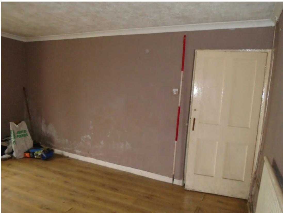
Figure 18 Room G3 looking south-west. Scale 1x2 m
