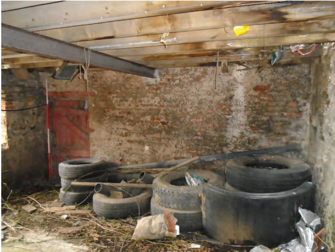
Figure 83 Room G3, facing south-west. Scale 1x2 m
