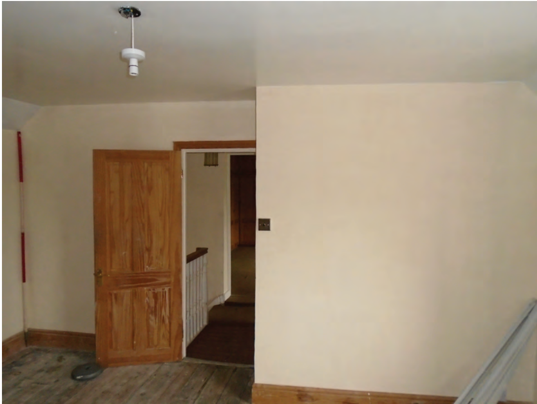
Figure 62 Room F8, facing north-east. Scale 1x2 m
