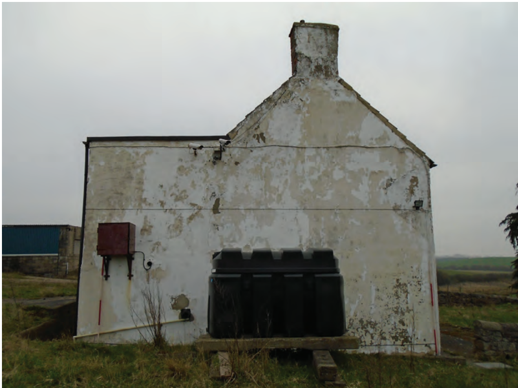
Figure 5 West elevation of Building A, facing east. Scale 2x2 m
