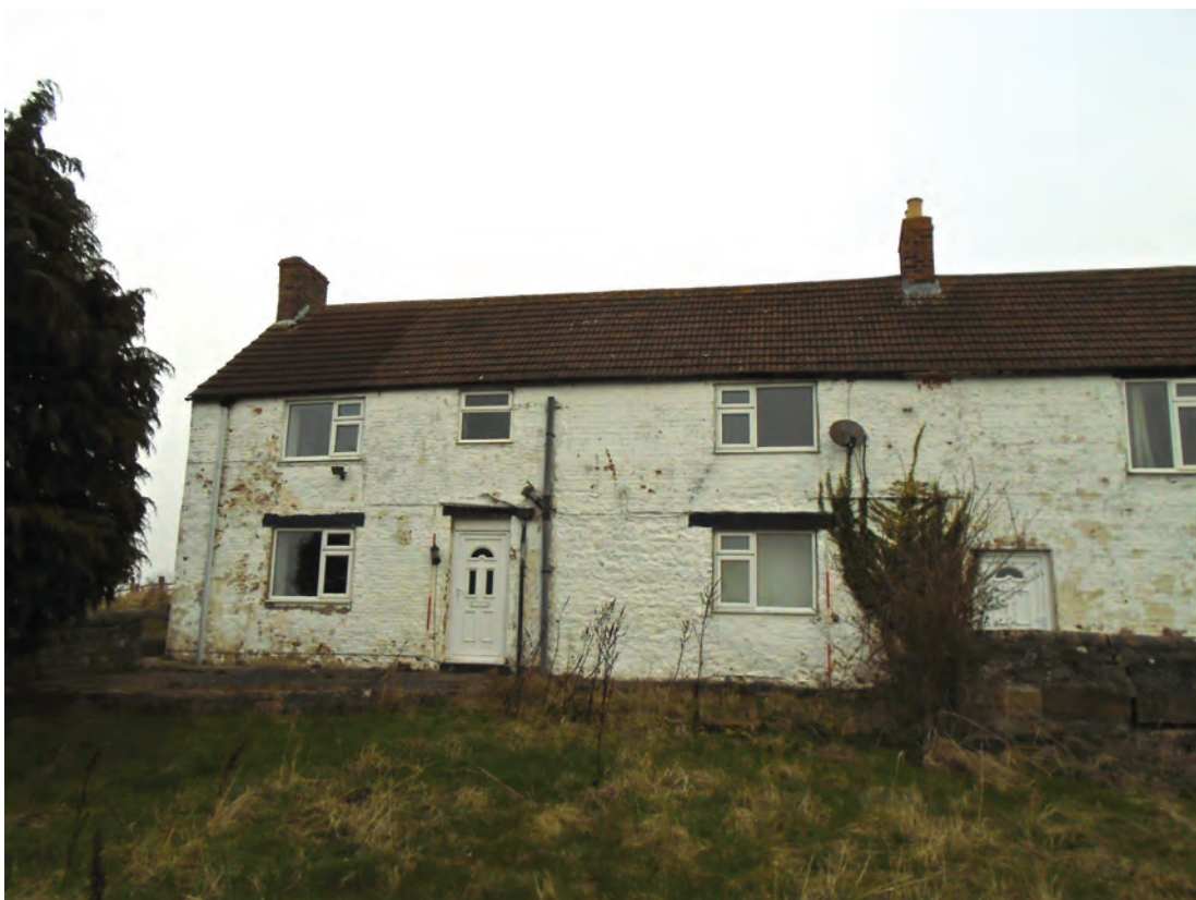
Figure 3 Western extent of south elevation of Building A. Scale 2x2 m
