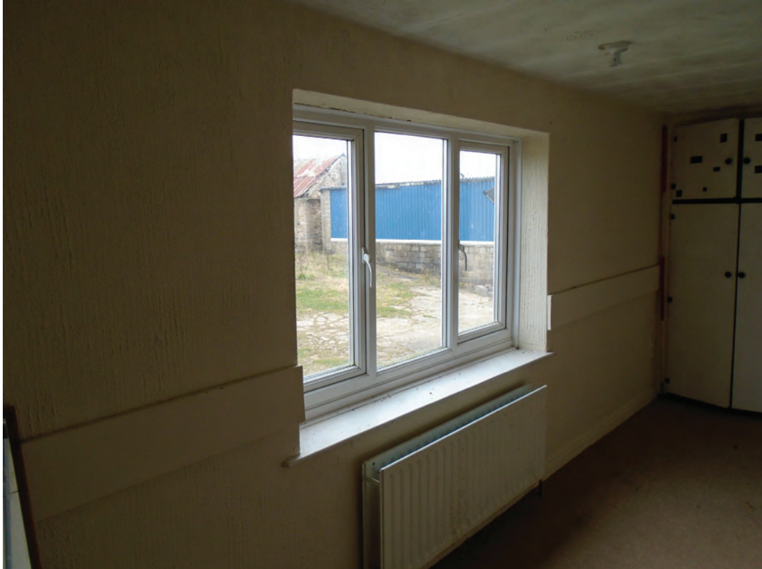
Figure 57 Room F6, facing north-east. Scale 1x2 m
