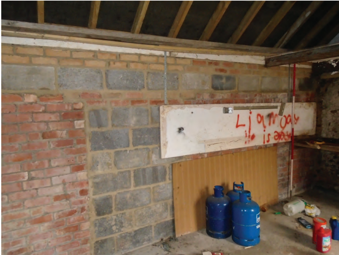
Figure 11 Room G1, facing south-west. Scale 1x2 m
