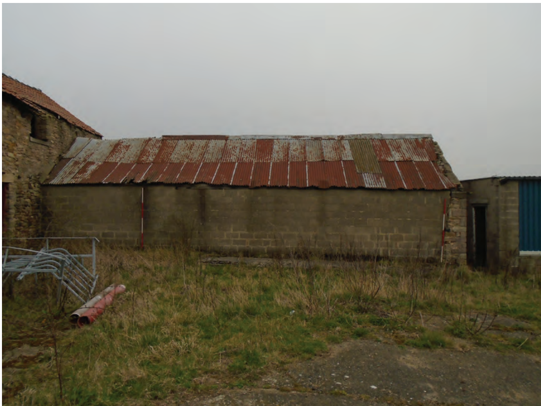
Figure 73 Building B, west elevation of single-storey barn. Scale 2x2 m
