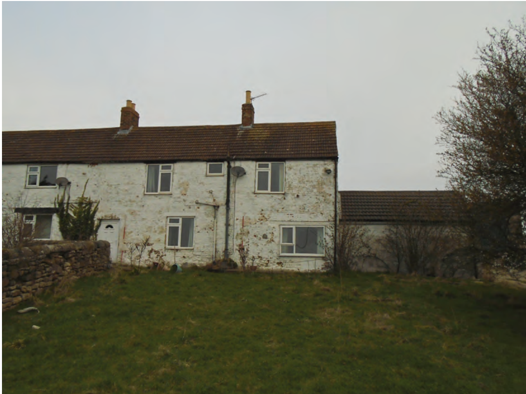
Figure 4 Eastern extent of south elevation of Building A. Scale 2x2 m
