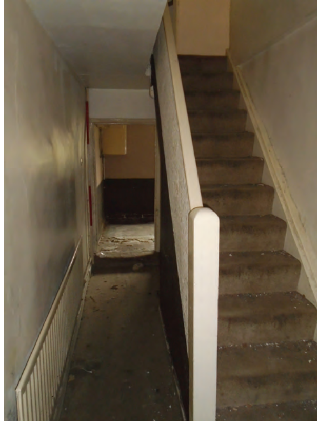
Figure 22 Room G6 looking north. Scale 1x2 m
