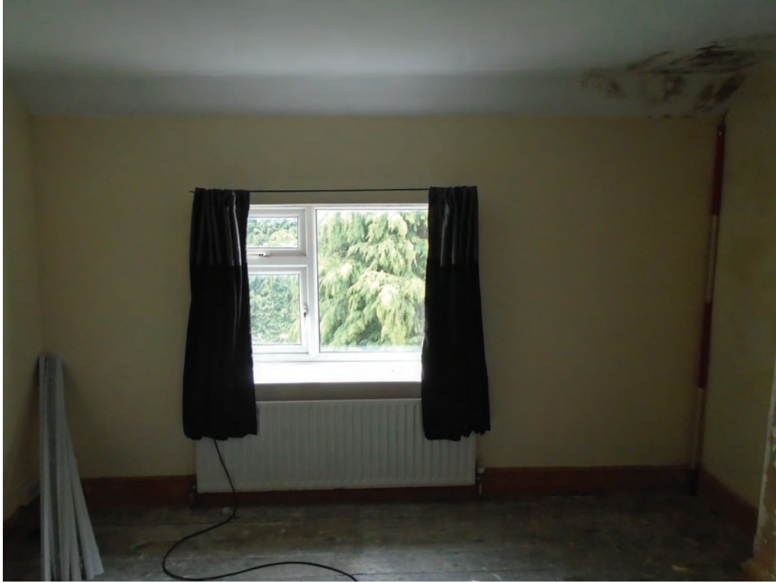
Figure 60 Room F8, facing south. Scale 1x2 m
