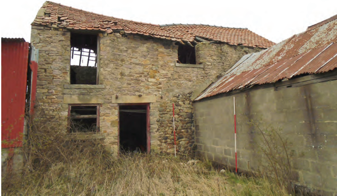
Figure 66 Building B south elevation, facing north-east. Scale 2x2 m
