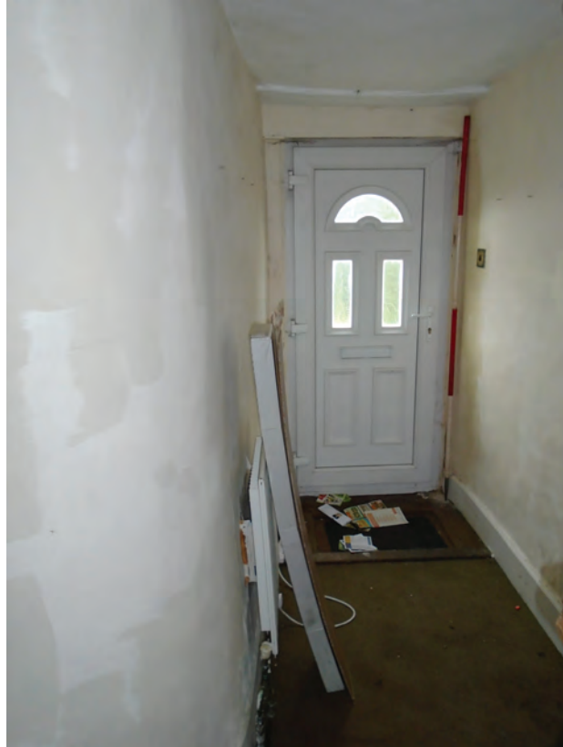
Figure 35 Room G10 looking south. Scale 1x2 m
