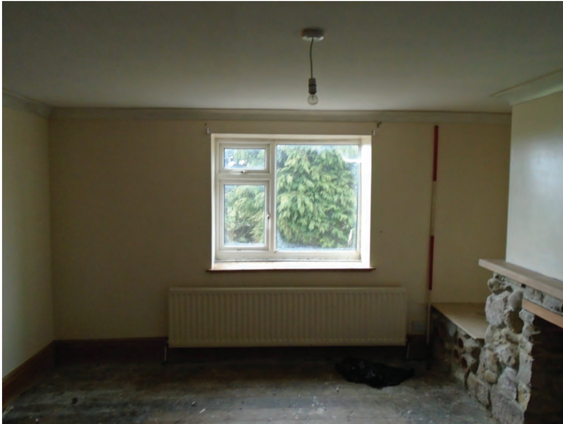
Figure 38 Room G11 looking south. Scale 1x2 m
