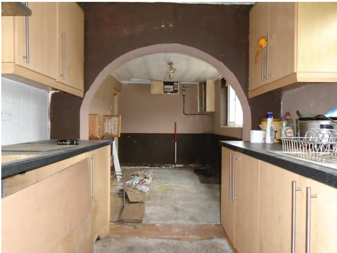
Figure 20 Room G4/G5 facing west. Scale 1x1 m
