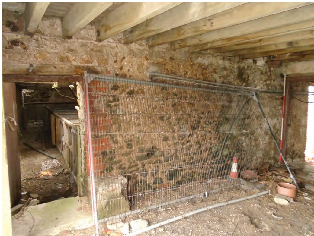
Figure 78 Room G2, facing south-west. Scale 1x2 m
