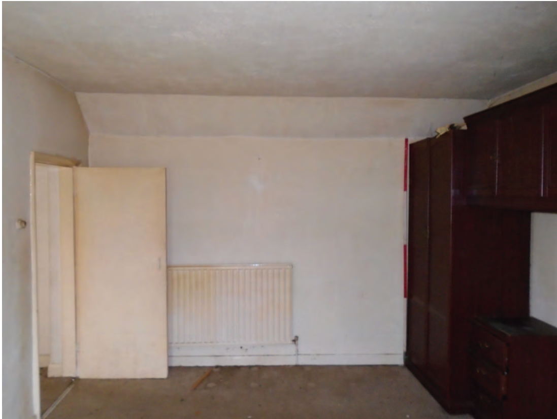
Figure 44 Room F1, facing north. Scale 1x2 m
