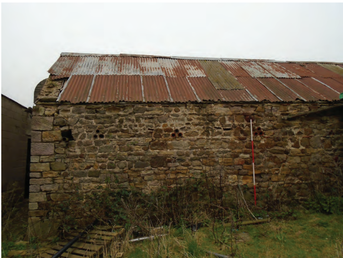
Figure 69 Building B, south extent of east elevation. Note 'breathers' for stock accommodation. Scale 1x2 m
