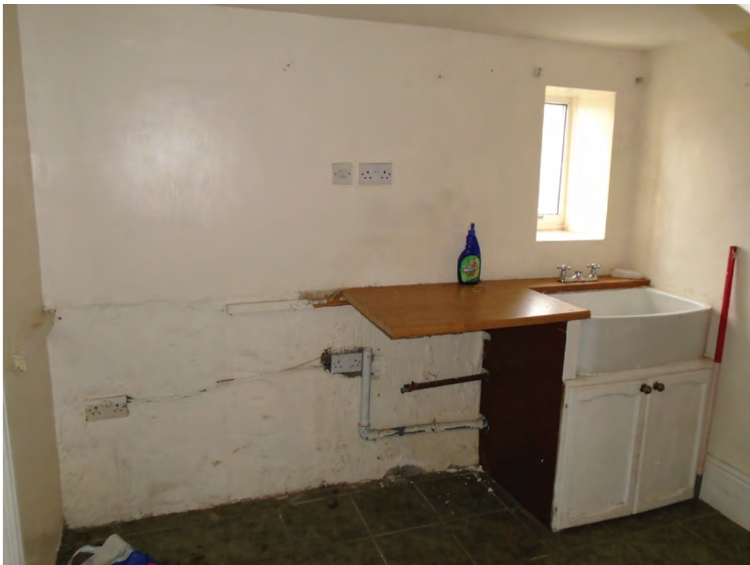
Figure 31 Room G9 looking north. Scale 1x1 m
