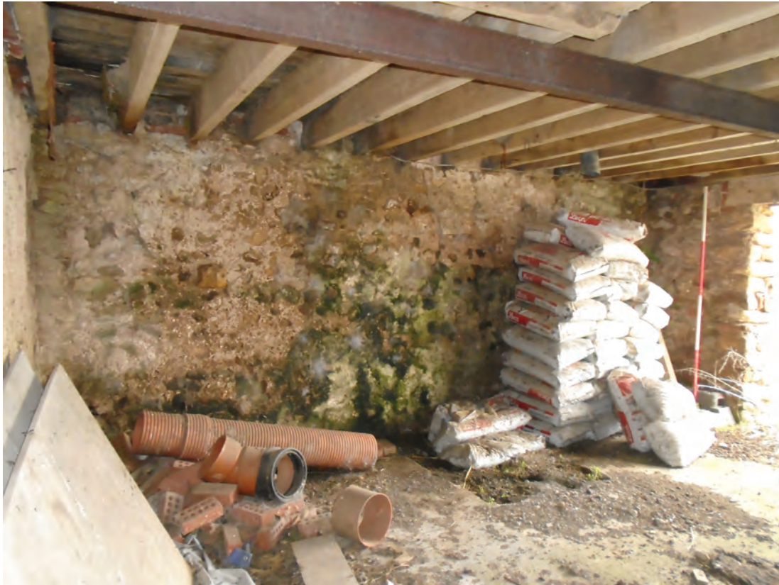
Figure 79 Room G2, facing north-east. Scale 1x2 m
