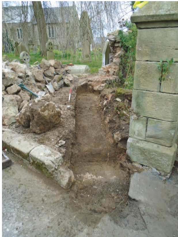
Figure 5 Completed excavation for new wall foundation, looking north. Scale 1x1 m
