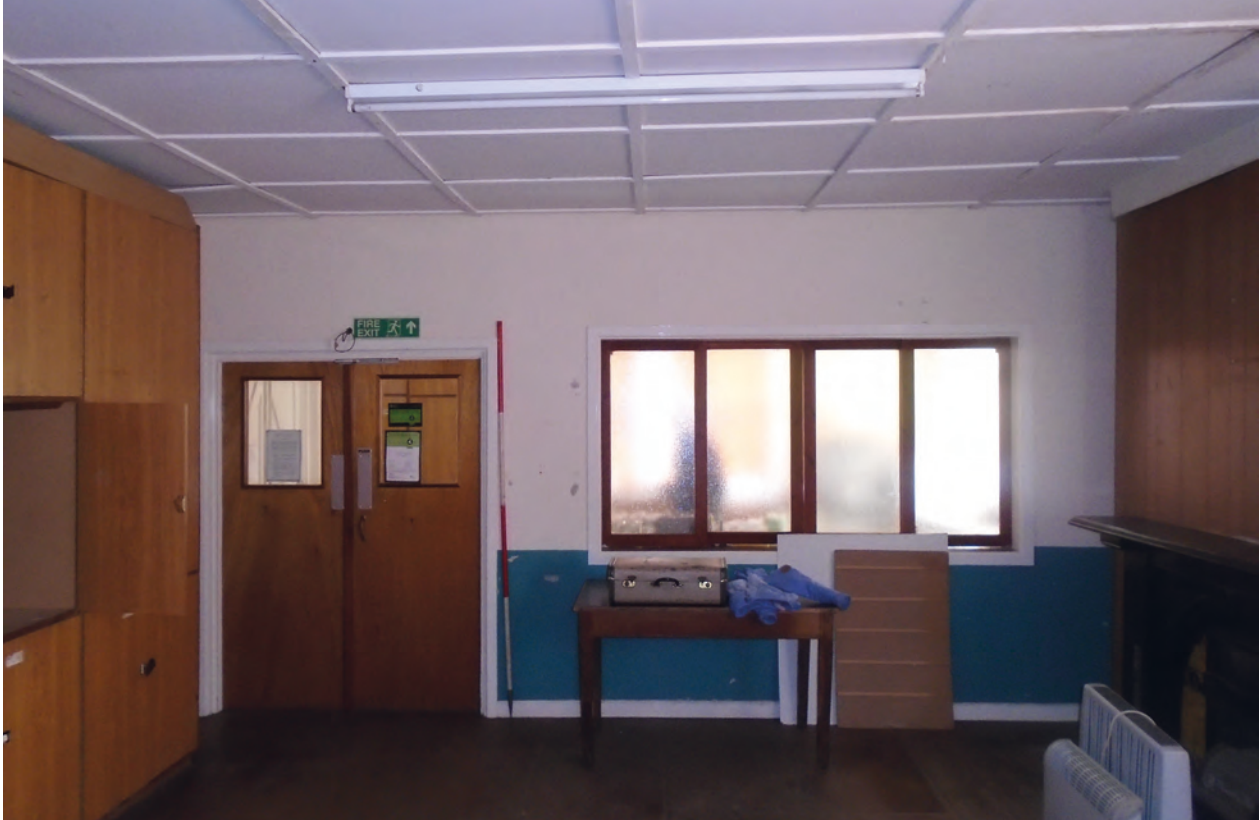
Figure 28 Room G7, facing north-east. Scale 1x2 m
