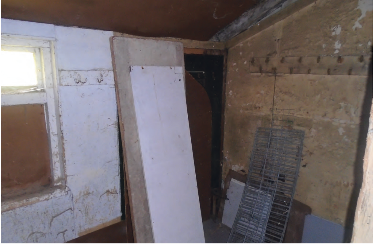
Figure 35 Room G9, facing west. No scale
