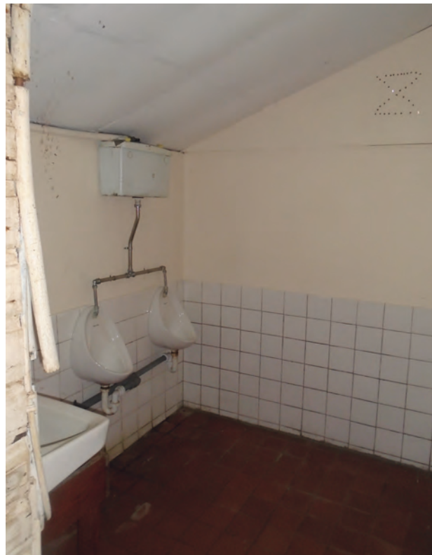
Figure 24 Room G6, looking north-west. No scale
