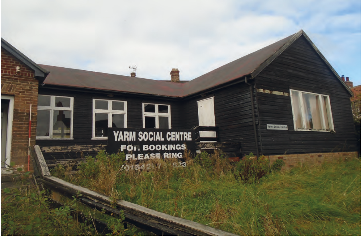
Figure 5 Western extent of north-east elevation. Scale 1x2 m
