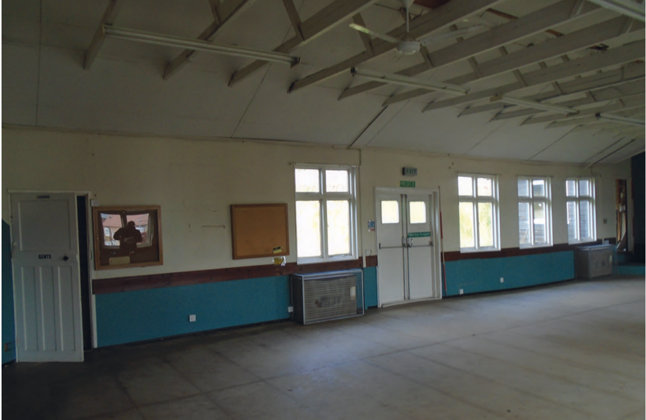
Figure 16 Room G2, south-west wall facing north-west. Scale 1x2 m
