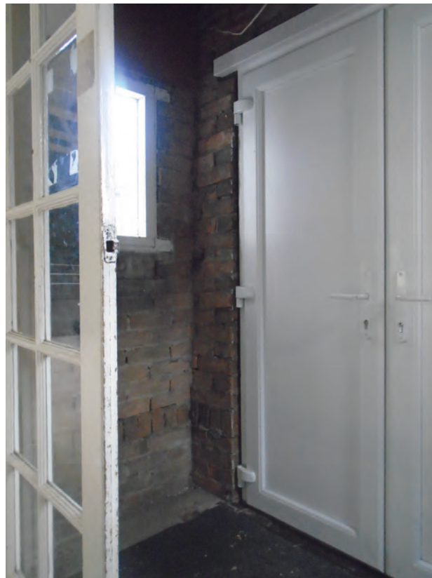
Figure 14 Room G1, facing north. No scale
