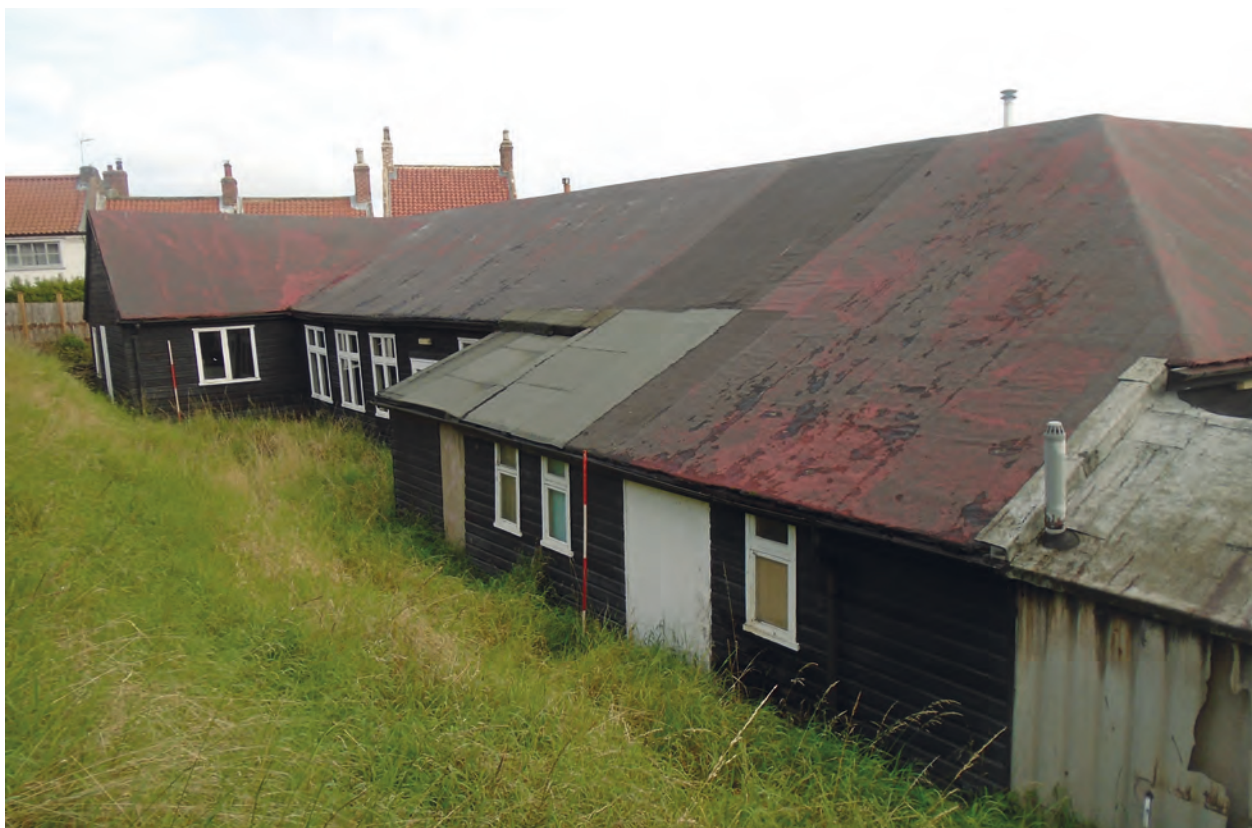
Figure 9 South-west elevation, facing north. Scale 2x2 m
