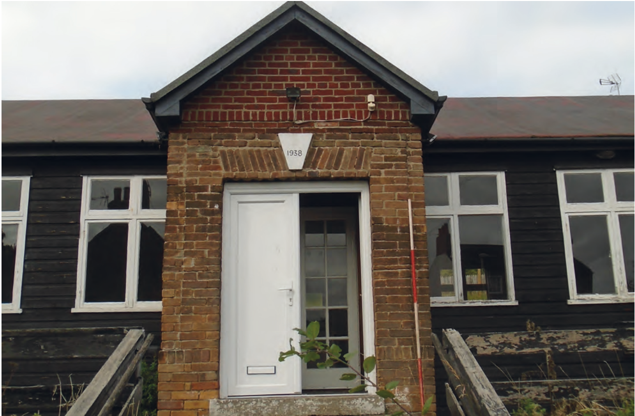
Figure 3 North-east elevation, central entrance porch. Scale 1x2 m
