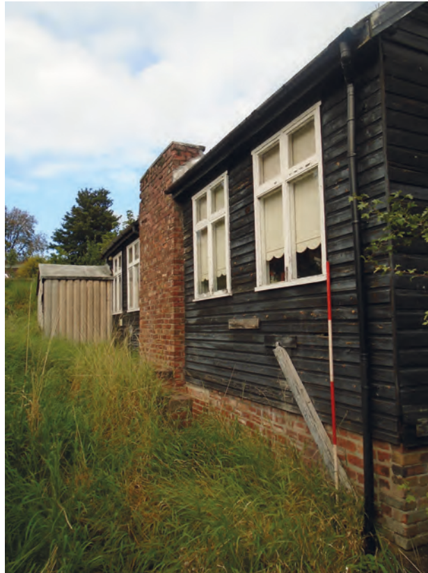
Figure 6 South-east elevation, looking west. Scale 1x2 m
