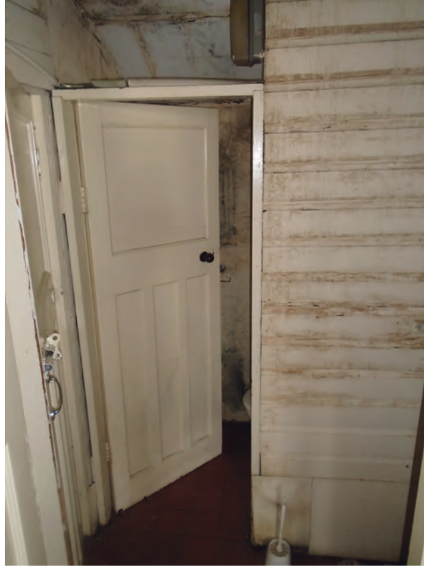
Figure 25 Room G6, central toilet cubicle. No scale
