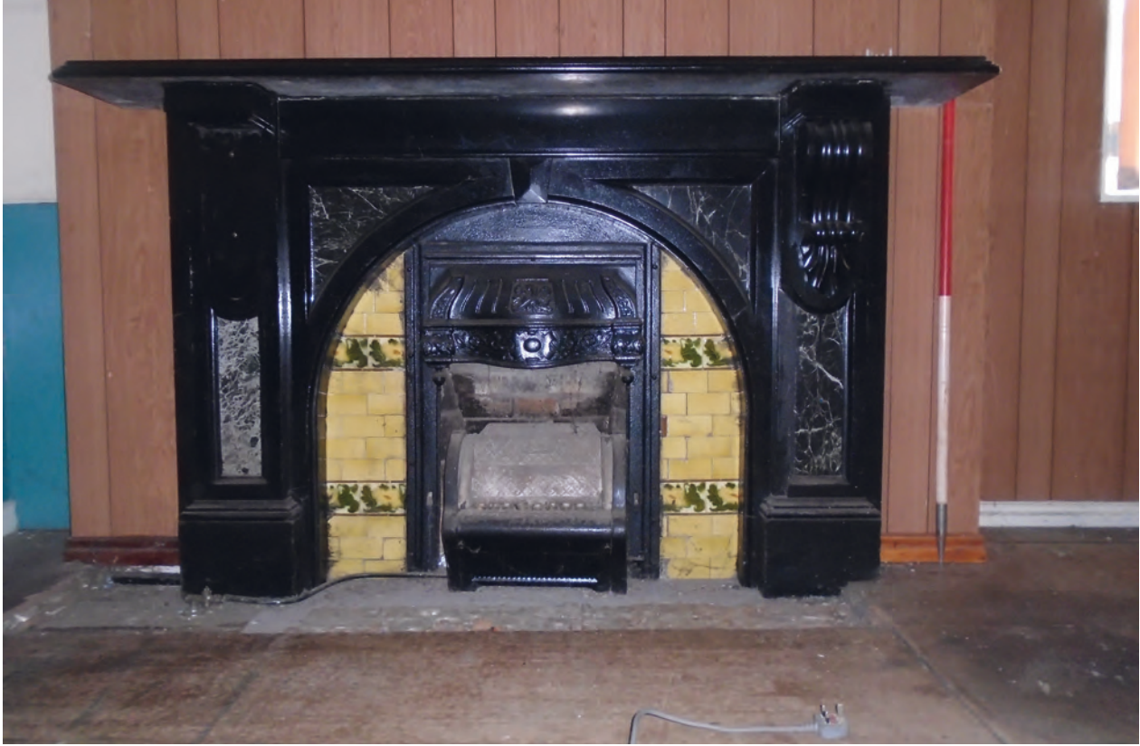
Figure 31 Detail of re-used Victorian fireplace. Scale 1x1 m
