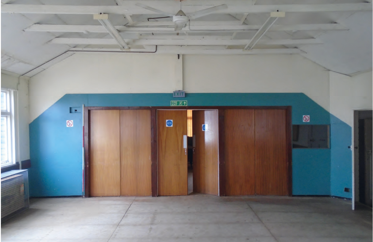
Figure 18 Room G2, south-east wall, including inserted doors. Scale 1x2 m
