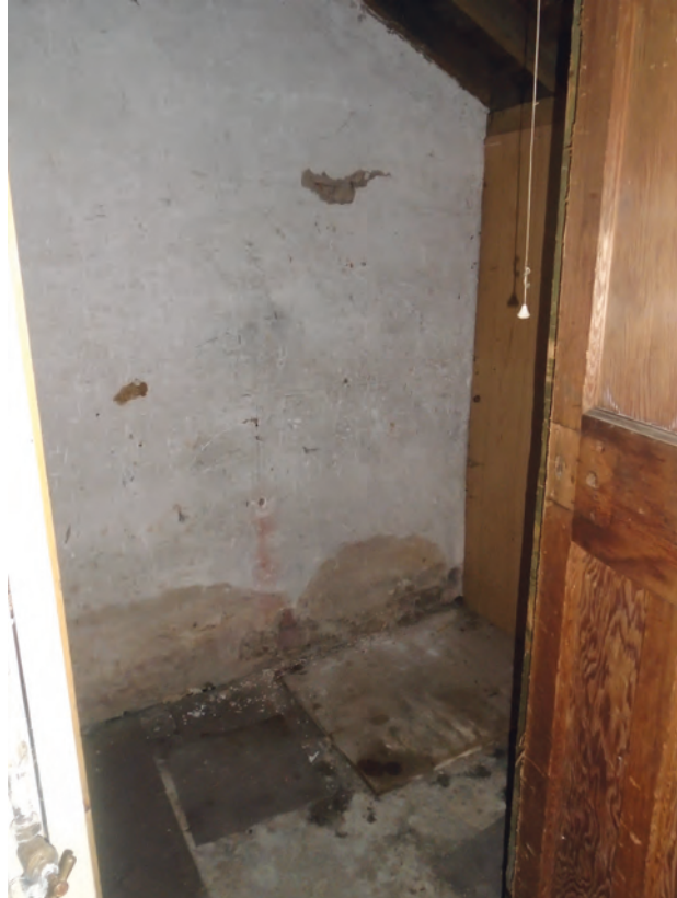
Figure 26 Room G6, looking south. No scale
