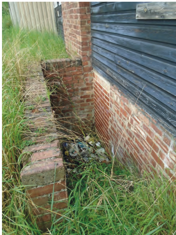
Figure 8 External stair access to cellar with blocked door. No scale
