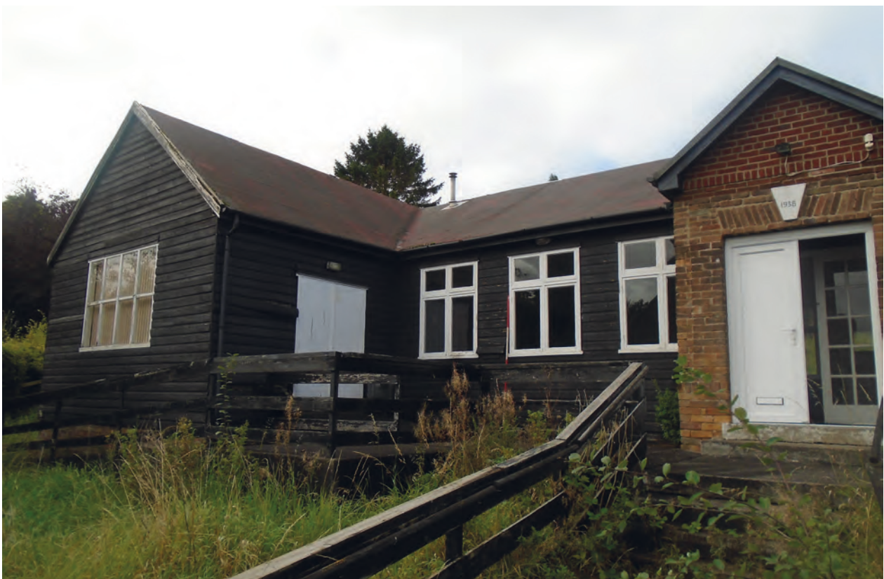
Figure 4 Eastern extent of north-east elevation. Scale 1x2 m
